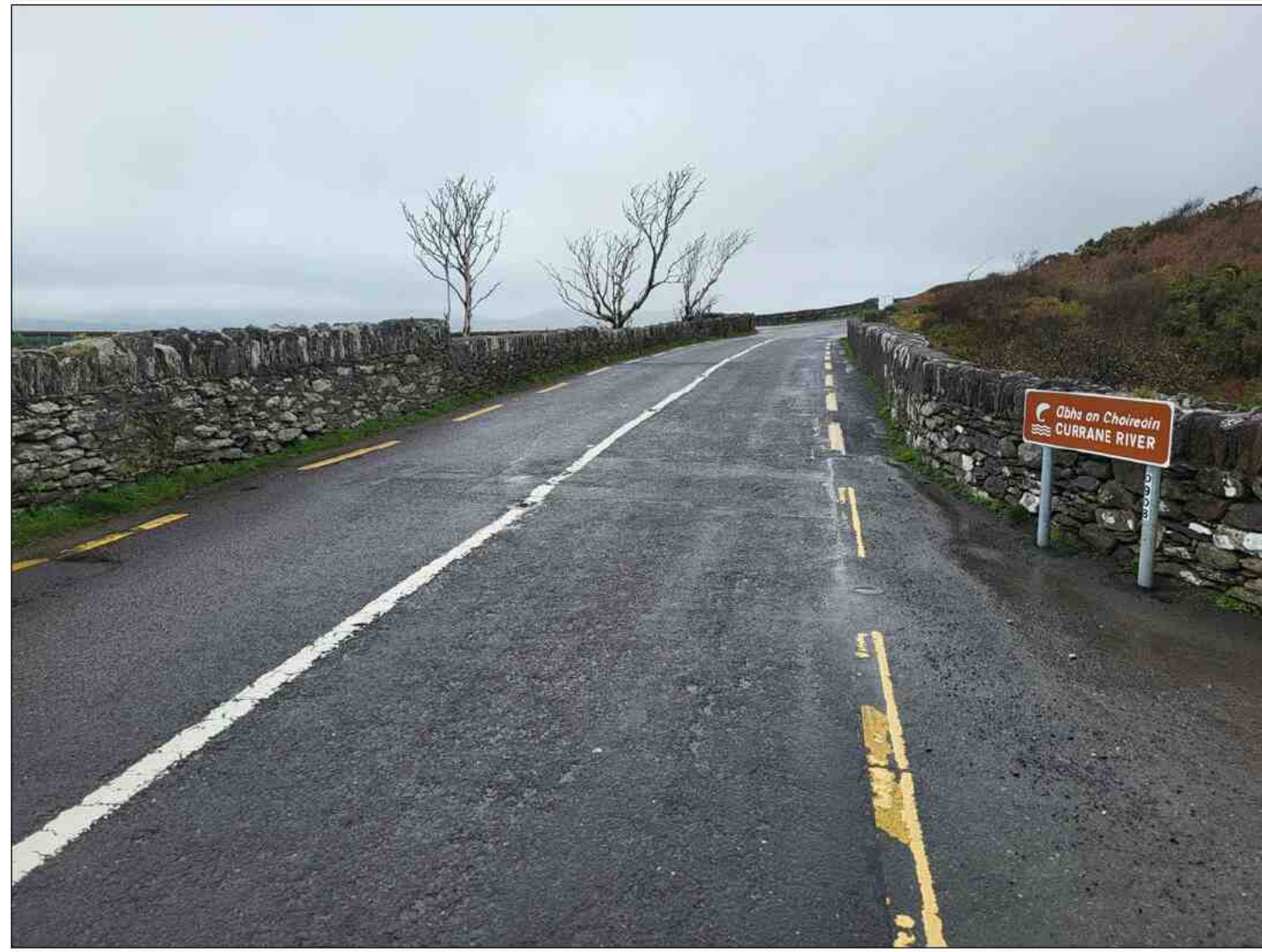
1. SOUTH APPROACH TO BRIDGE LOOKING NORTH
