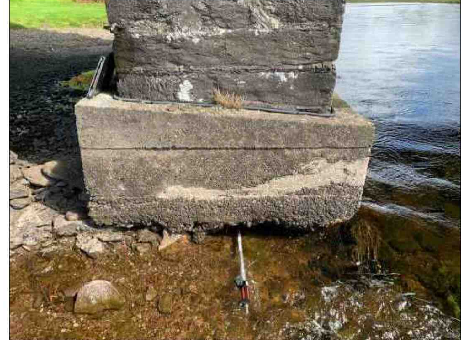
9. UNDERMINING OF THE SCOUR PROTECTION AT THE WEST END OF THE NORTHERN PIER
