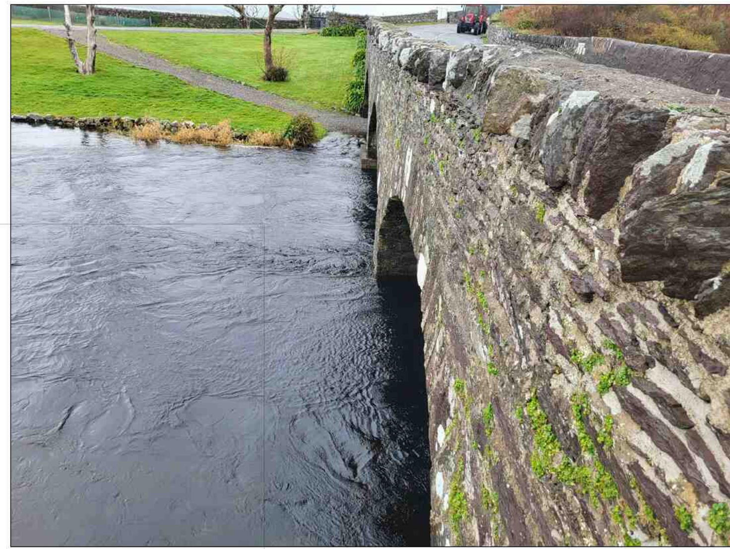
5. WESTERN SPANDREL WALL
