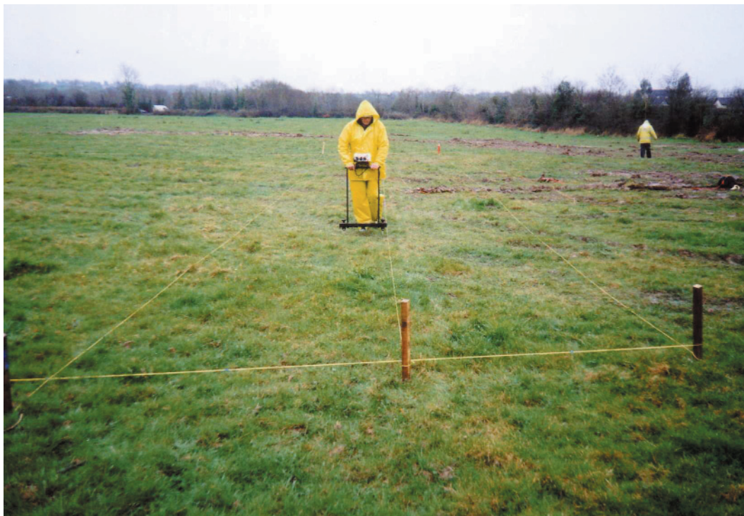
Geophysical survey using an electrical resistance metre on the N25 Waterford Bypass (Tramore House Regional Design Office)
