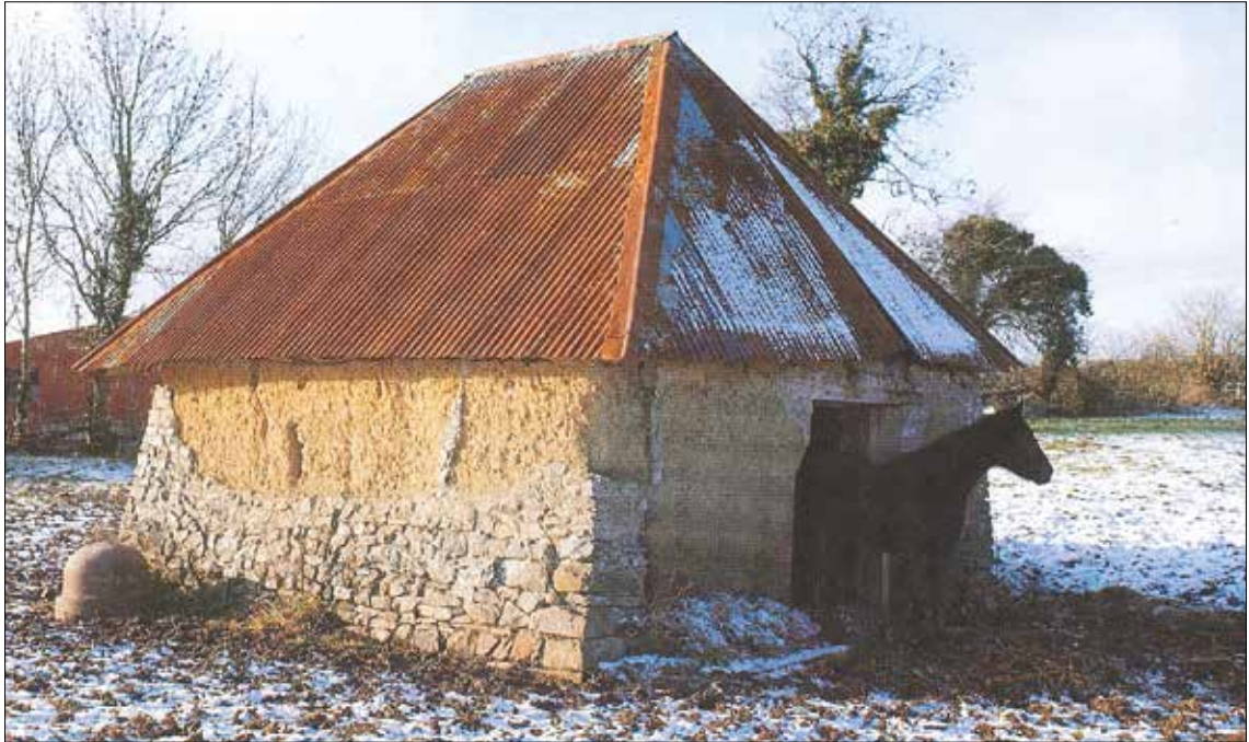
Illus. 3.5.2—A 19th-century example of a cob-built house with stone foundations near Enfield, Co. Meath (Walter Pfeiffer). Where walls are constructed entirely of cob, little physical evidence would survive the passage of centuries.
