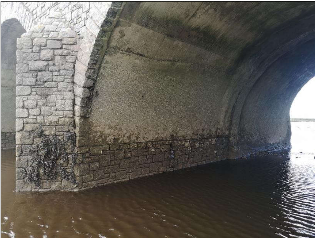
Plate 1.10 View of the north face of pier 1.
