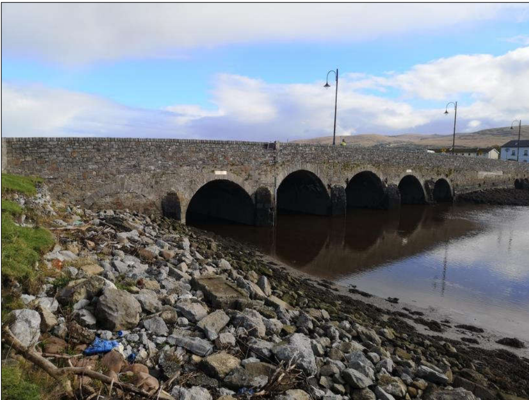
Plate 1.22 View of the west elevation.
