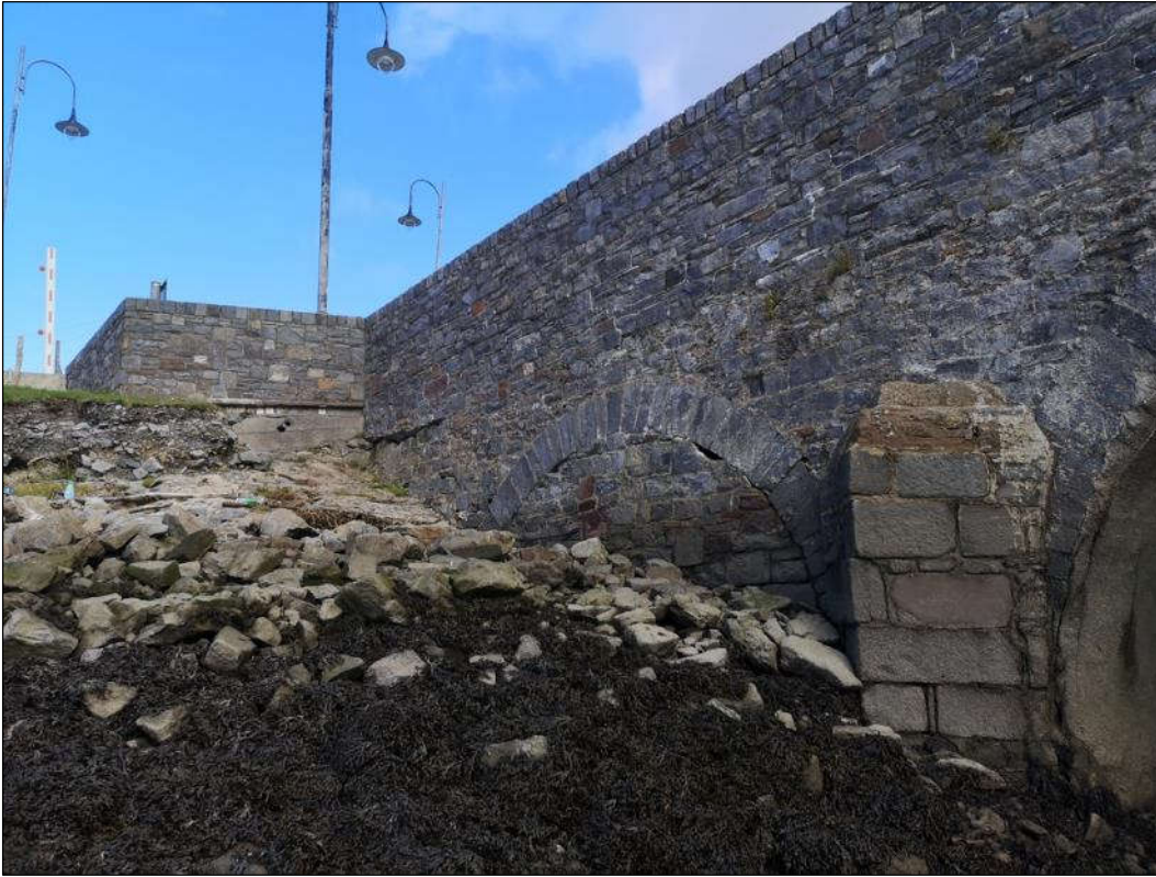
Plate 1.5 View of the NW wing wall and infilled north span.
