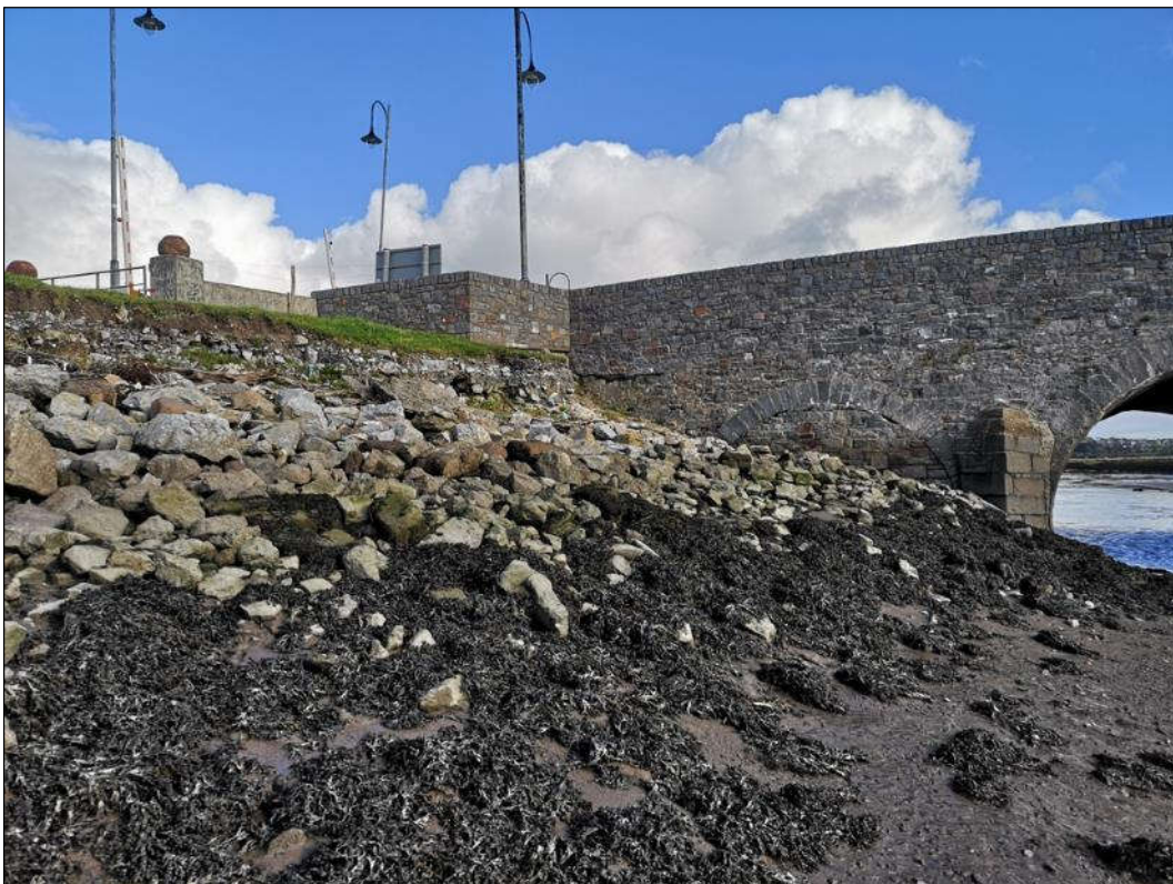
Plate 1.4 View of the NW embankment.
