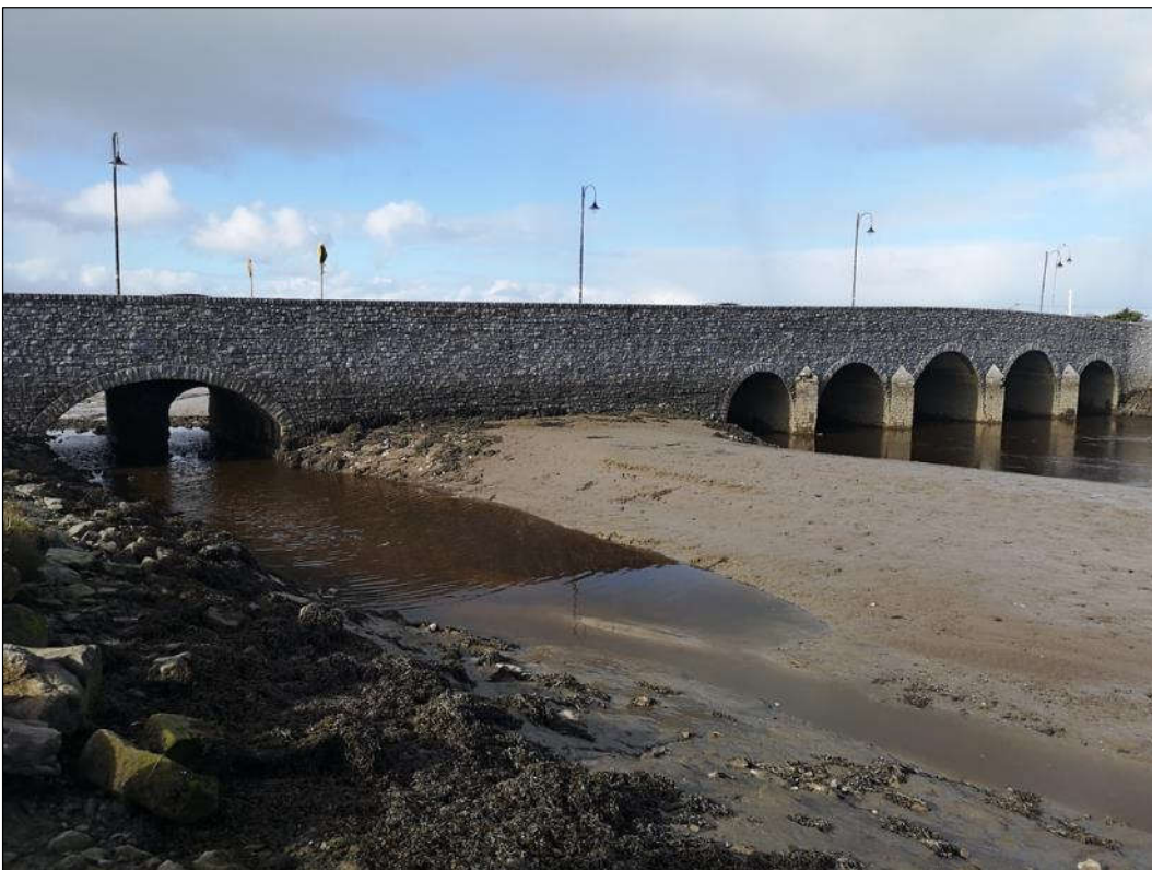
Plate 1.20 View of the riverbed at the east elevation.
