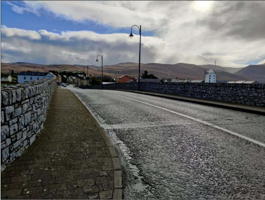
Plate 1.1 Bridge surface looking south.
