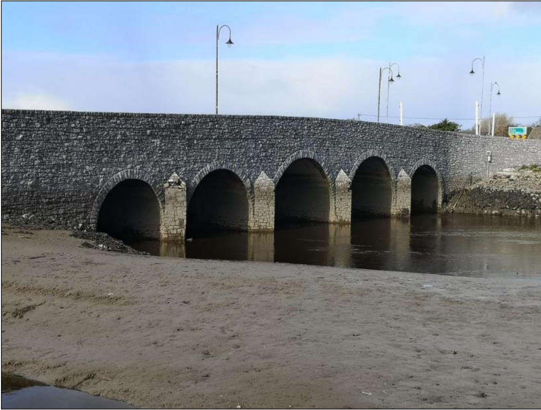
Plate 1.21 View of the east elevation.
