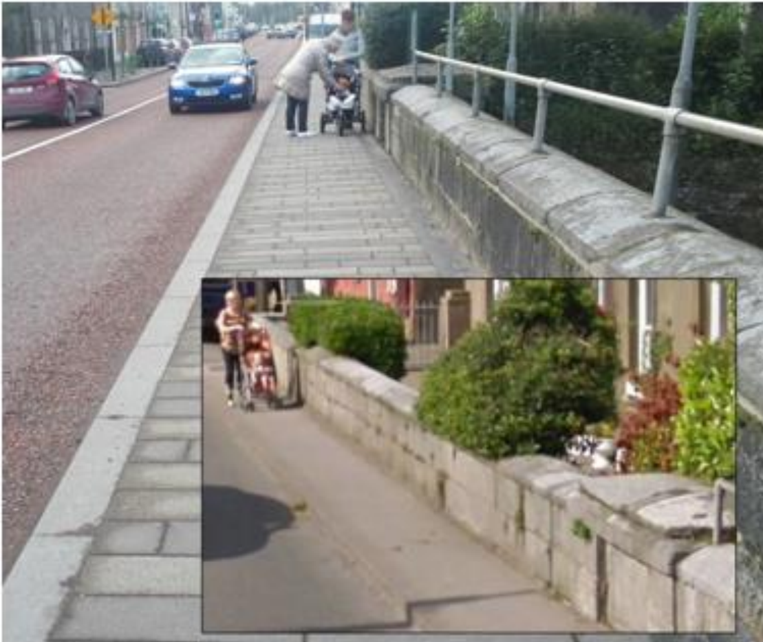
Figure 5.1 Footpath widening Killishan, Co. Cork
