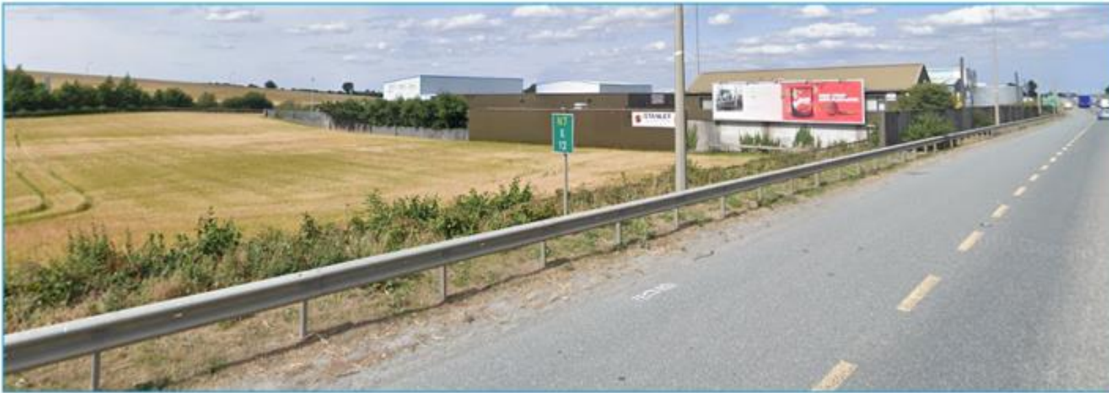
Figure 3-13 - Inaccessible Stop opposite Blackchurch Inn, in verge behind safety barrier
