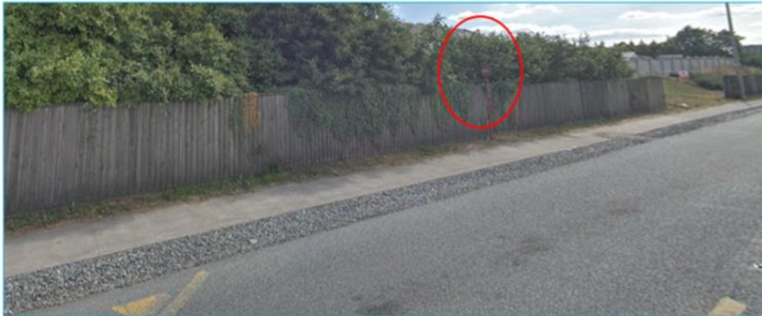
Figure 3-10 - Bus Stop location in hard shoulder at end of Rathcoole merge lane
