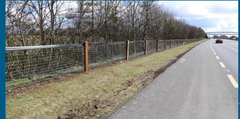
Repairs to Mesh fence following collision
