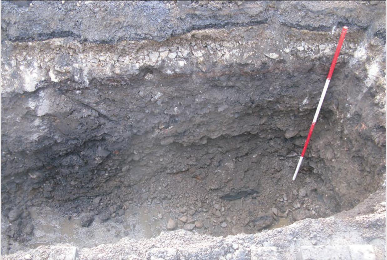
Plate 5 - ST-123, N facing section of trench showing gravel embankment (028)
