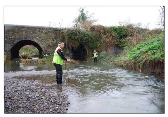
**Plate 5:** Working-shot of diver undertaking riverbed survey along downstream side of Lissenhall Bridge, northern flow-channel of Broadmeadow River. Note: diver tethered to counteract against river-flow.
