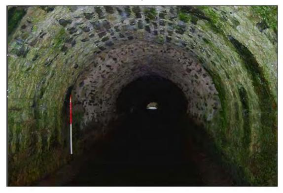
Plate 78: East-facing view though Arch no. 2 showing transition between the upstream (Phase 3) and middle section (Phase 1) at Balheary Bridge, Feature 3 (1m scale).
