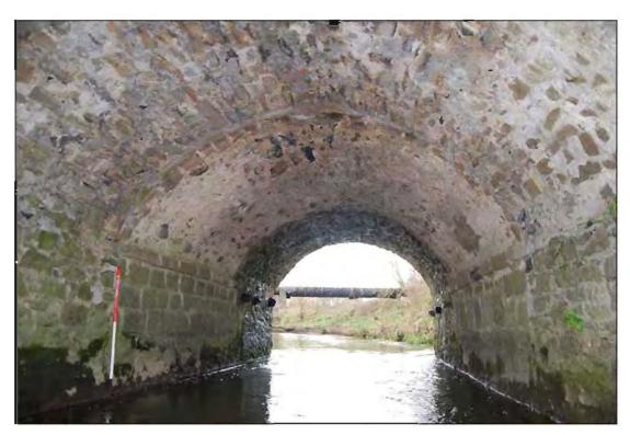
Plate 39: West-facing view of arch-walls and intrados from Arch no. 2, Lissenhall Bridge, Feature 1 (1m scale).
