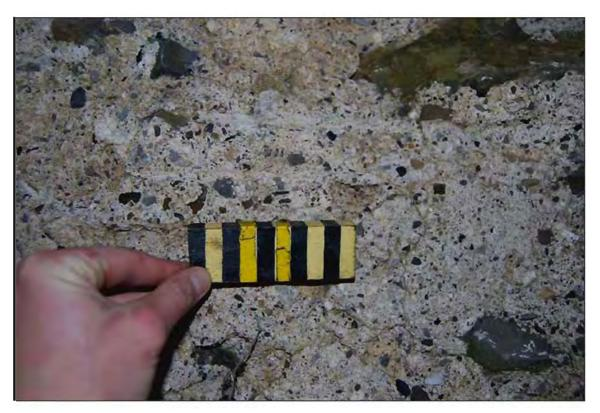
**Plate 41:** Detail shot of coarse mortar covering the intrados of the mid-section of Lissenhall Bridge. (10cm scale).
