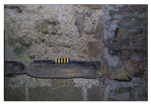
Plate 45: North-facing view across lintel forming at top of arch-wall on north side of the midsection of Arch no. 2, Lissenhall Bridge, Feature 1 (10cm scale).
