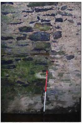
Plate 28: Transition-point between mid-section (Phase 1) and upstream section (Phase 2), north side of Arch no. 5 (1m scale).
