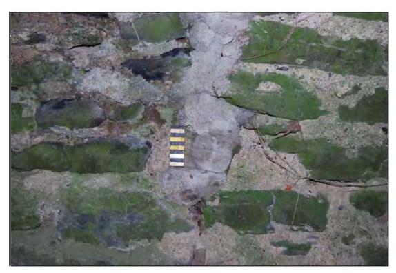
Plate 53: Detail shot of intrados transition-point between the upstream section (Phase 2) and the middle section (Phase 1) from Arch no. 1, Lissenhall Bridge, Feature 1 (10cm scale).
