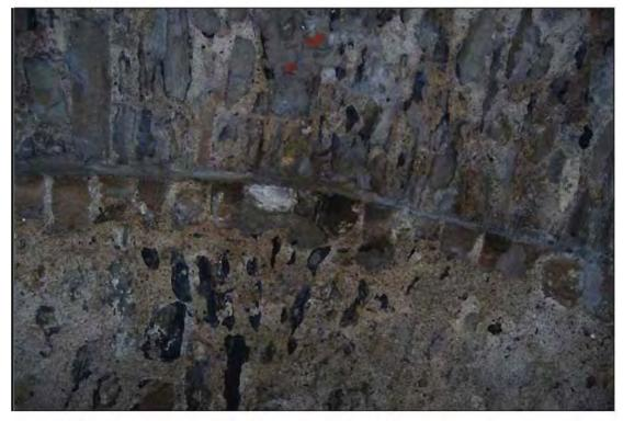
Plate 54: Detail shot of intrados transition-point between the middle section (Phase 1) and the downstream section (Phase 2) within Arch no. 2, Lissenhall Bridge (Feature 1).
