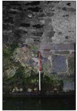
Plate 22: Transition-point between mid-section (Phase 1) and upstream section (Phase 2), north side of Arch no. 2 (1m scale).
