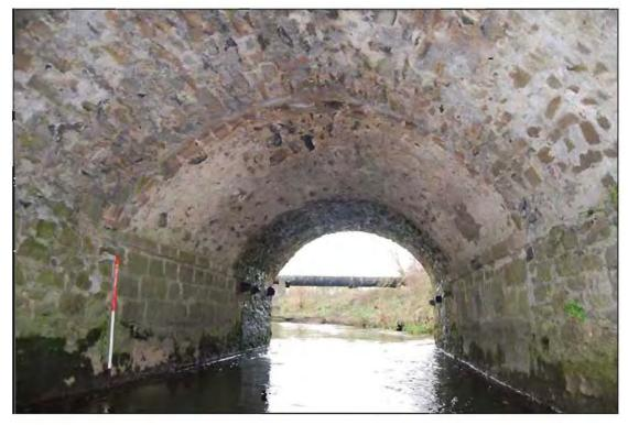
**Plate 56:** West-facing view across arch-ceiling (intrados) of **Arch no. 2**, Lissenhall Bridge (Feature 1). Note: differing composition of intrados and protruding arch-stones from downstream side of mid-section (1m scale).
