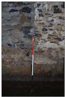
Plate 73: Transition-point between mid-section (Phase 1) and downstream section (Phase 2), north side of Arch no. 1 (1m scale).
