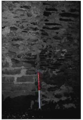
Plate 38: Transition-point between mid-section (Phase 1) and downstream section (Phase 2), north side of **Arch no. 5** (1m scale).
