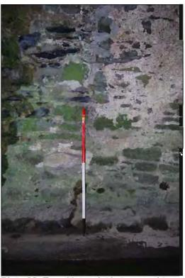
Plate 32: Transition-point between mid-section (Phase 1) and downstream section (Phase 2), north side of **Arch no. 2** (1m scale).
