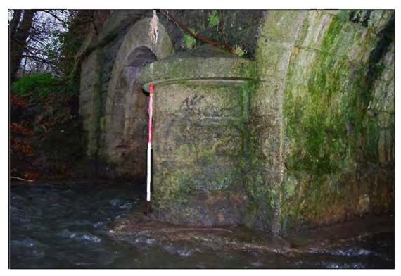
Plate 81: North-facing view of semi-circular cutwater located between Arch nos. 1 and 2 on upstream side of Balheary Bridge, Feature 3 (1m scale). Note: concrete underpinning of bridge structure.
