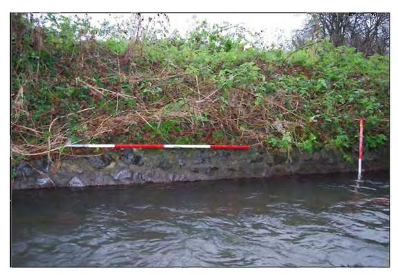
Plate 85: North-facing detail shot of revetment wall (Feature 5, Section 1) located along north side of the river (1m vertical and 2m horizontal scale).
