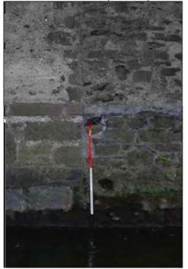
Plate 21: Transition-point between mid-section (Phase 1) and upstream section (Phase 2), south side of Arch no. 2 (1m scale).
