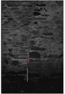
Plate 37: Transition-point between mid-section (Phase 1) and downstream section (Phase 2), south side of Arch no. 5 (1m scale).
