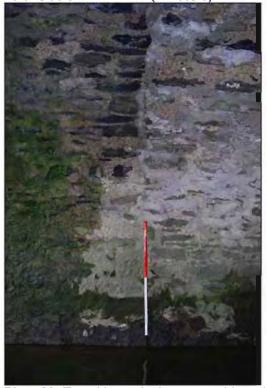
Plate 26: Transition-point between mid-section (Phase 1) and upstream section (Phase 2), north side of Arch no. 4 (1m scale).
