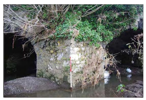
**Plate 49:** East-facing view of Cutwater no. 3, located between Arch nos. 3 and 4, Lissehanll Bridge, Feature 1 (1m scale).
