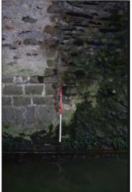
Plate 34: Transition-point between mid-section (Phase 1) and downstream section (Phase 2), north side of Arch no. 3 (1m scale).
