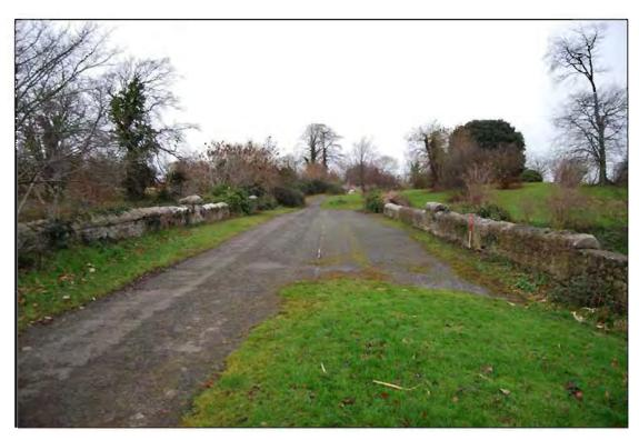
Plate 11: North-facing view of upper surface of Lissenhall Bridge (Feature 1) showing residue of tarmacadam from the R127 (1m scale).
