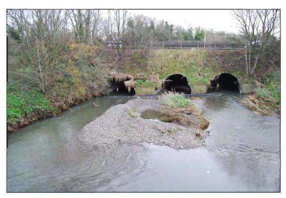
Plate 1: East-facing view of downstream side of Lissenhall Bridge showing pebble island and three-arched culvert that accommodates the N1 Link-Road (1m horizontal and 2m vertical scale).
