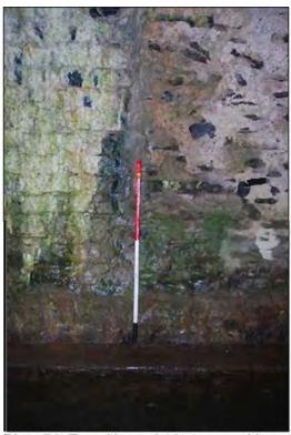
Plate 74: Transition-point between mid-section (Phase 1) and upstream section (Phase 3), north side of Arch no. 2 (1m scale).
