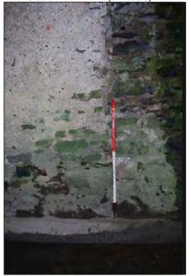
Plate 30: Transition-point between mid-section (Phase 1) and downstream section (Phase 2), north side of **Arch no. 1** (1m scale).
