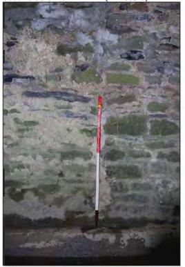
Plate 29: Transition-point between mid-section (Phase 1) and downstream section (Phase 2), south side of Arch no. 1 (1m scale).
