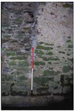
Plate 31: Transition-point between mid-section (Phase 1) and downstream section (Phase 2), south side of Arch no. 2 (1m scale).
