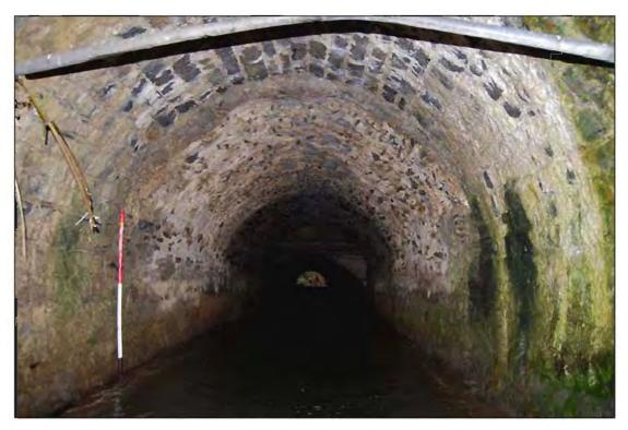
Plate 77: East-facing view though Arch no. 1 showing transition between the upstream (Phase 3) and middle section (Phase 1) at Balheary Bridge, Feature 3 (1m scale).
