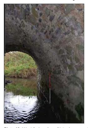
**Plate 46:** West-facing view of intrados on north side of **Arch no. 4**, showing bulge located across the arch-ceiling of the phase 1 mid-section, Lissenhall Bridge, Feature 1 (1m scale).
