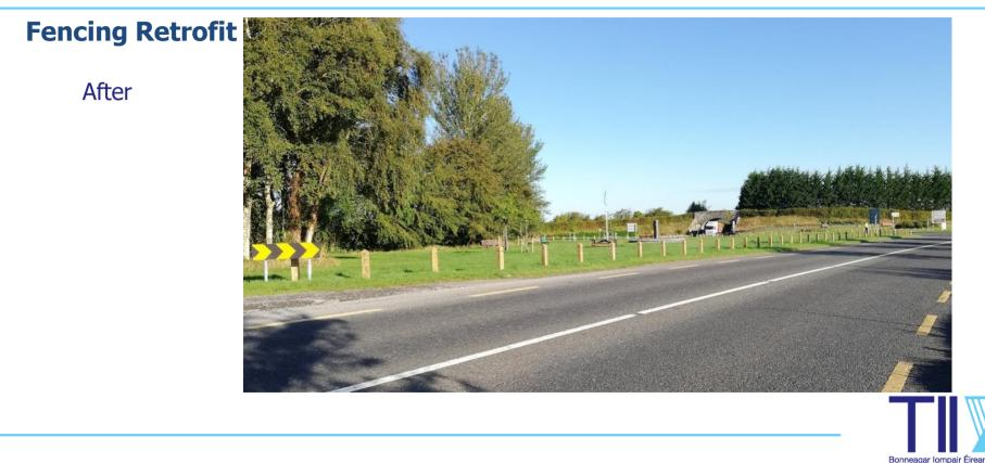
**Example** - RSI 33109 N80 Co. Laois. Unforgiving roadside hazard. Removal of post and fence rail and replaced with a timber post and tension mesh fence in accordance with RCD 300/21.
