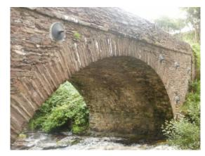
Tie-bars and Pattress plates prevent overturning of parapet and spandrel wall
