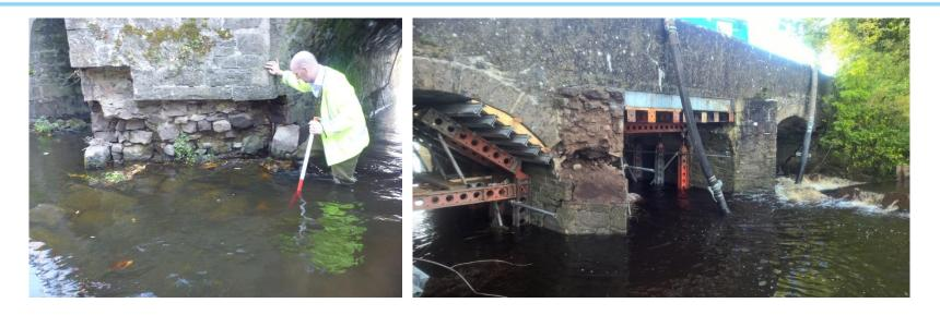
Bridges with shallow foundations are most susceptible to scour damage from erosion of the river bed
