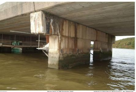
Concrete delamination, concrete cracking, rust staining, leachate staining, dampness, failed expansion joints, marine environment, vulnerable half-joint detail
