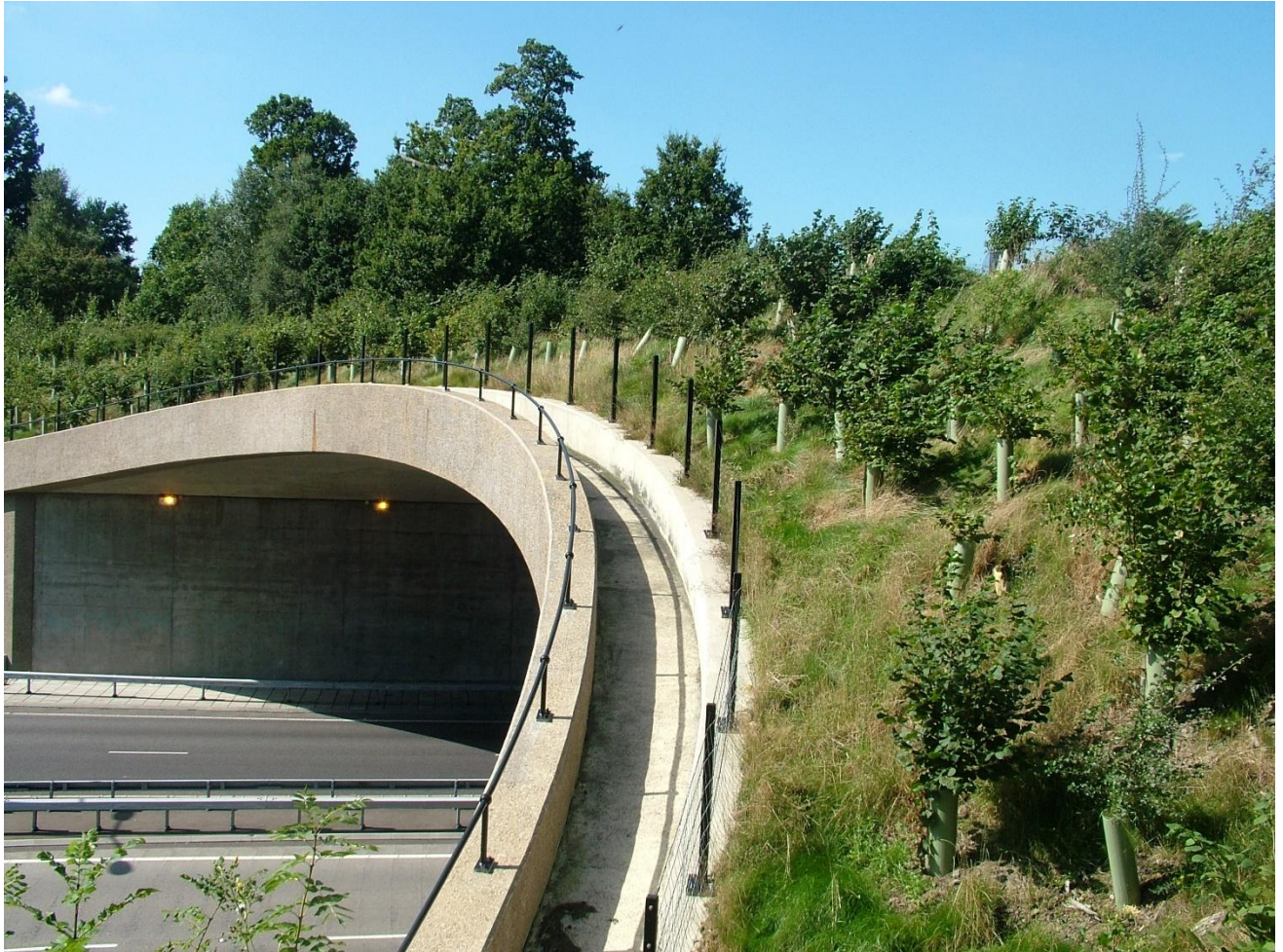
Plate 2: Green Bridge to mitigate the effects of habitat fragmentation (A21 Lamberhurst Bypass, Kent, UK)
