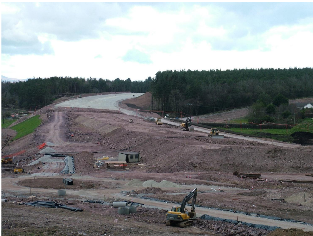
Plate 1: The M8 Rathcormac - Fermoy Bypass under construction, showing habitat fragmentation (Ballybrack Wood, Fermoy) in 2004
