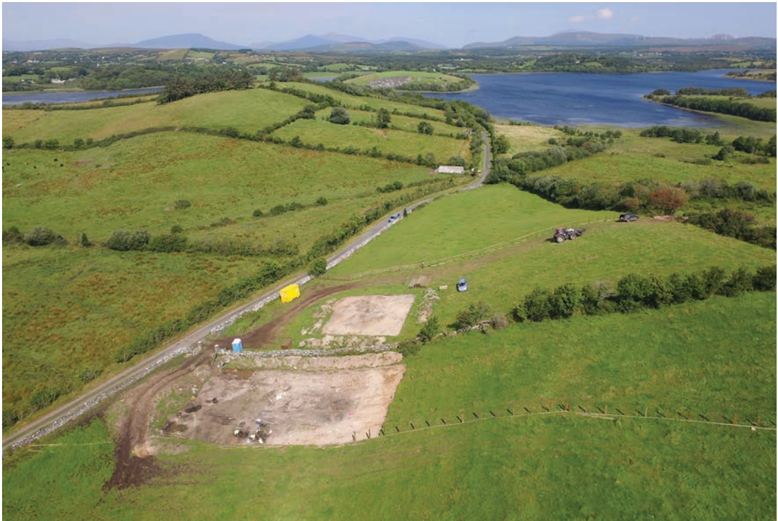
Illus. 1.7 Excavating Claggarnagh East 4/5 (foreground) and 6 between two drumlins, looking north to Islandeady Lough, Co. Mayo (Firefly Photography for Mayo County Council).
