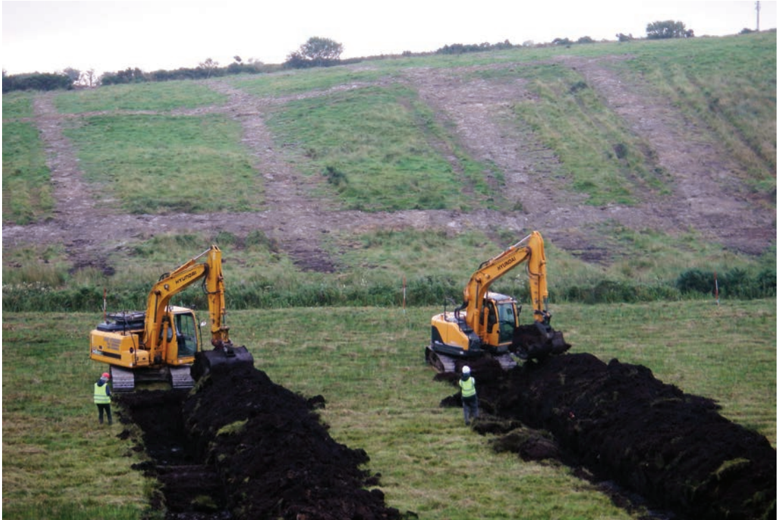
Illus. 1.3 Test-excavations in Drumneen with trenching in peaty topsoil in progress in the foreground and completed, backfilled trenches on the hillslope in the background (ACSU Ltd).
