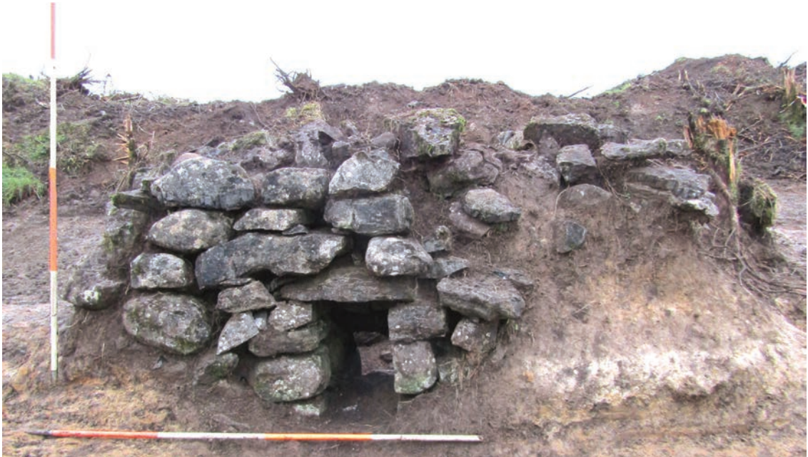
Illus. 5.15 Liscromwell 1. This simple lime kiln, built with local limestone rubble, is a typical example of the small kilns that became ubiquitous in rural Ireland in the early modern period (ACSU Ltd).
