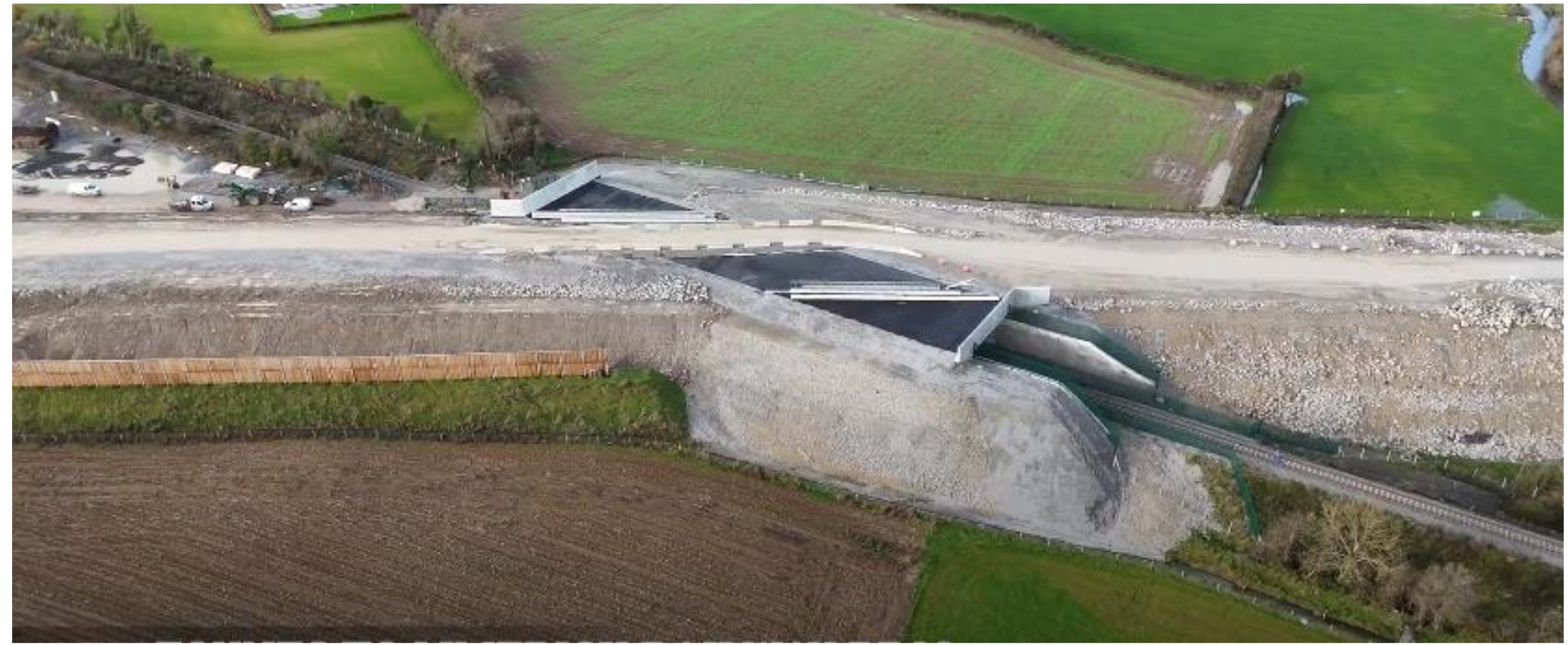
Railbridge RB02 Gortnagrour Adare - Lot1
