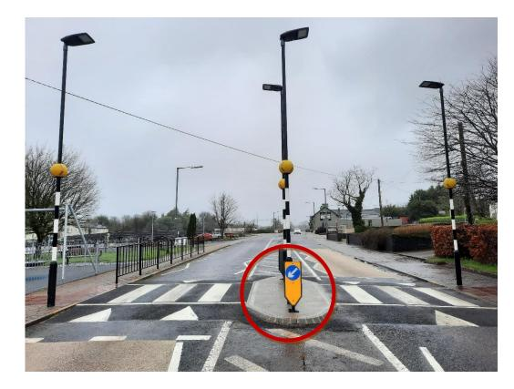
Central Island is greater than 2.00m wide? Should it be a refuge? Tactile paving? How should a pedestrian/driver interpret it?
