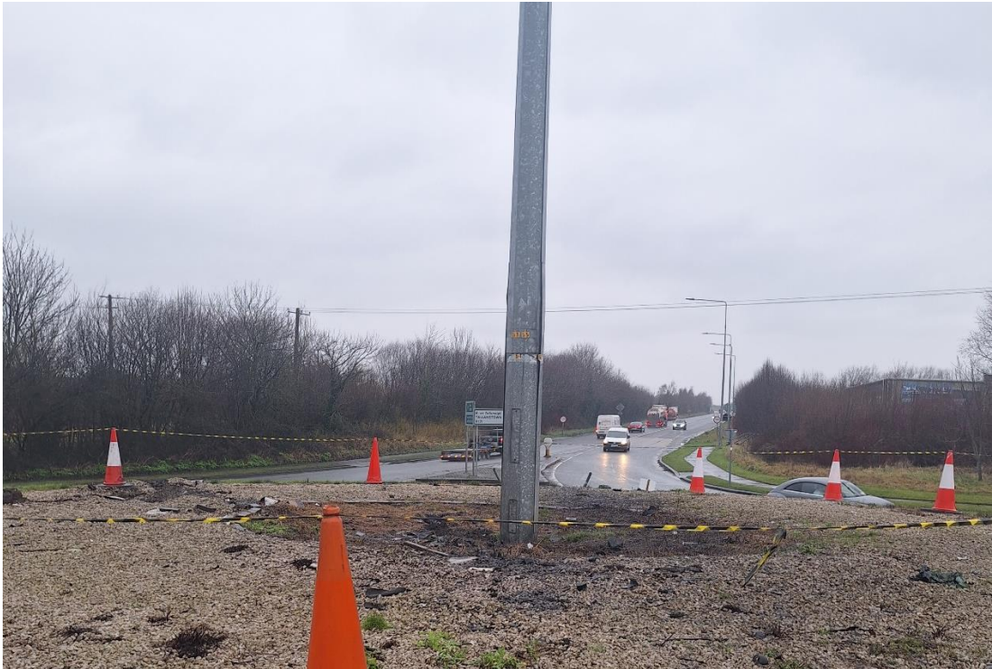
High Mast impact damage (LH-N02-701.00)
