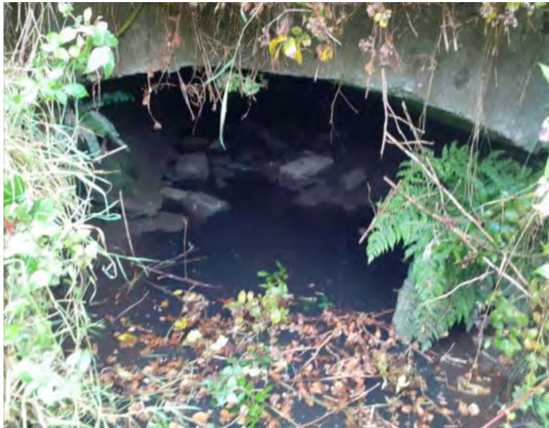
Figure 3-1 - Downstream of the Culvert
