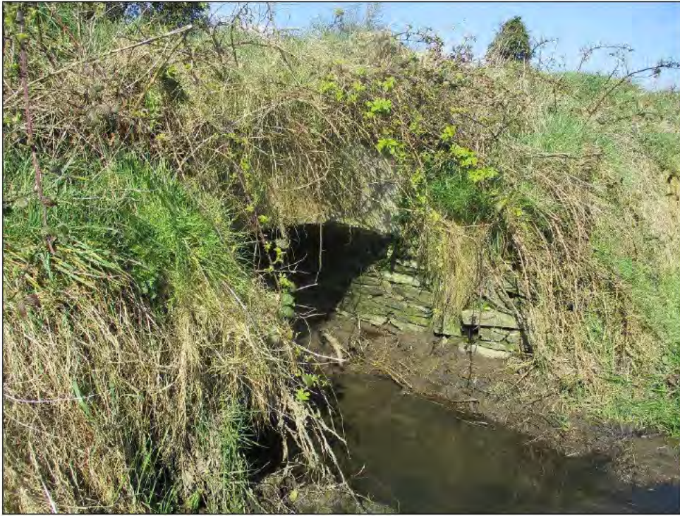
Plate 4.2 - View of Cavan Bridge (culvert).
