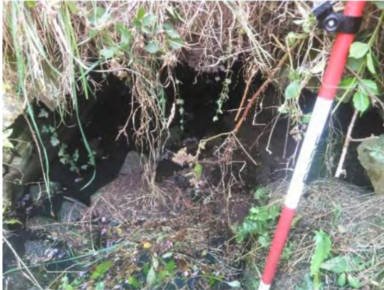
Figure 3-2 - Upstream of the culvert
