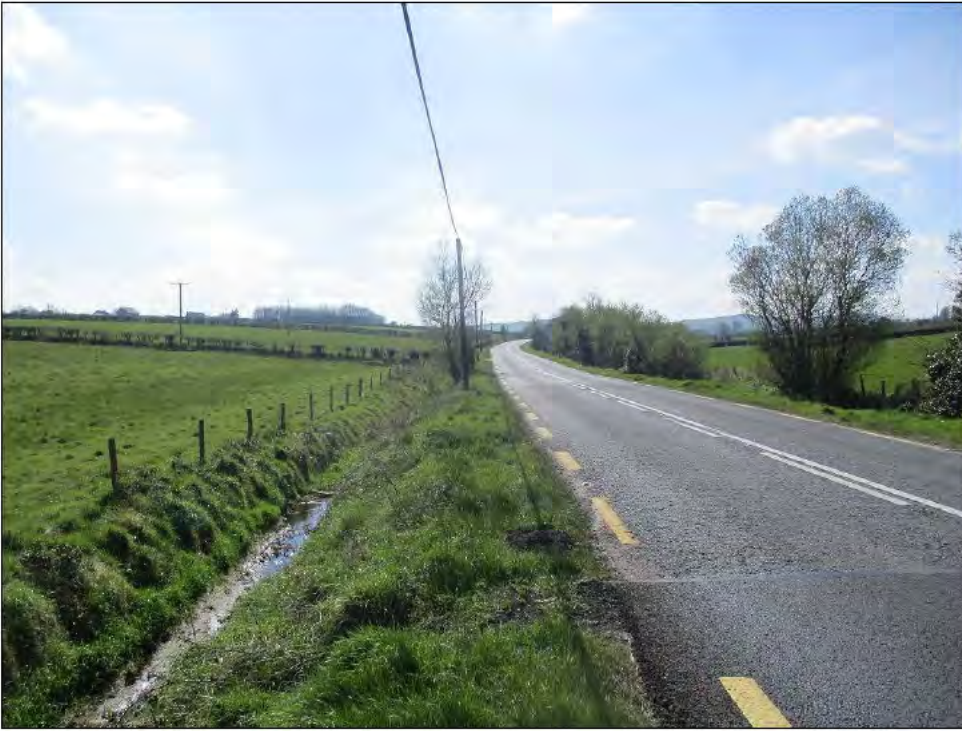
Plate 4.6 - Cavan Bridge Culvert and stream/ditch to the left and the N14 to the right.
