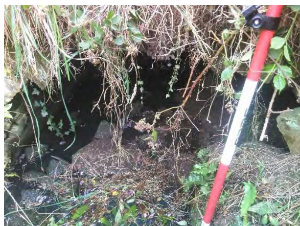
Figure 3-2 – Cavan culvert upstream
