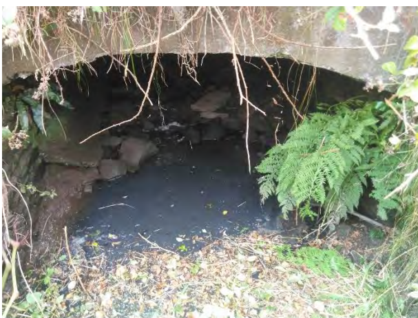
Figure 3-1 - Cavan culvert downstream
