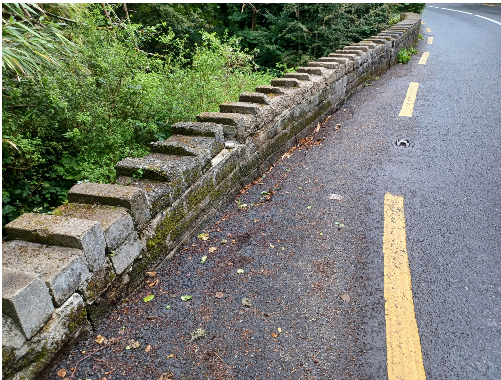
Figure 2: Damaged section of the parapet and carriageway to be repaired at Moyard Bridge (GC-N59-017.00).
