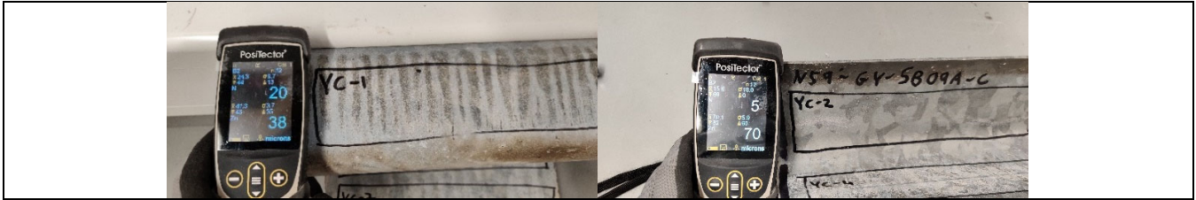
Figure 1: Example of measurement on area '1' (left) and '2' (right) for crash barrier labelled 'N59-GY-SB09A'.
