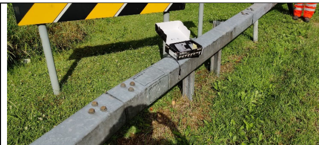
Figure 1: Testing site on N4 Carrick-on Shannon (east)
