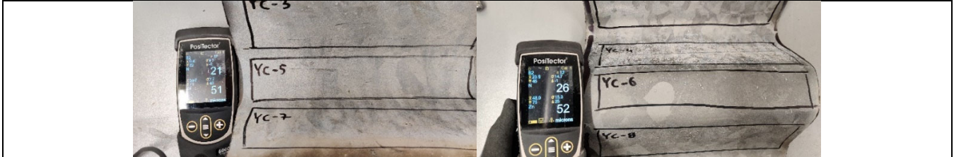
Figure 3: Example of measurement on area '5' (left) and '6' (right) for crash barrier labelled 'N59-GY-SB09A'.
