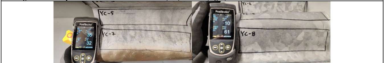
Figure 4: Example of measurement on area '7' (left) and '8' (right) for crash barrier labelled 'N59-GY-SB09A'.
