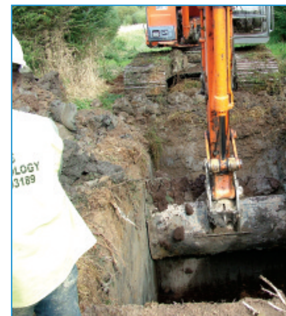
Archaeologist monitoring the excavation of a test pit in alluvium along the route of the Limerick Southern Ring Road (Phase II).
