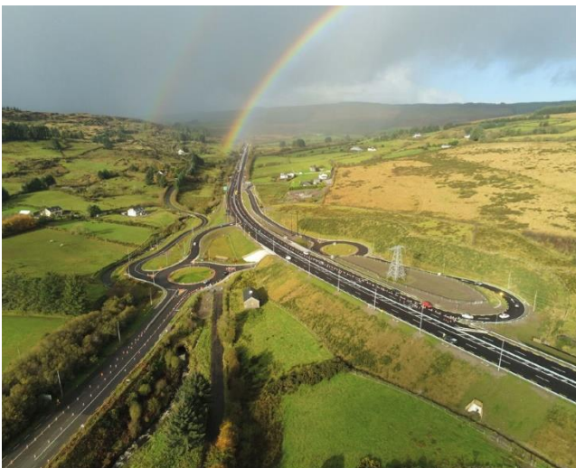
Figure 6 N22 Baile Bhúirne Junction on the Bypass
