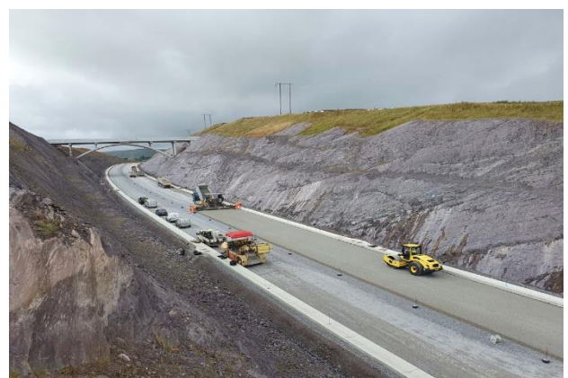
Figure 7 Construction of the N22
