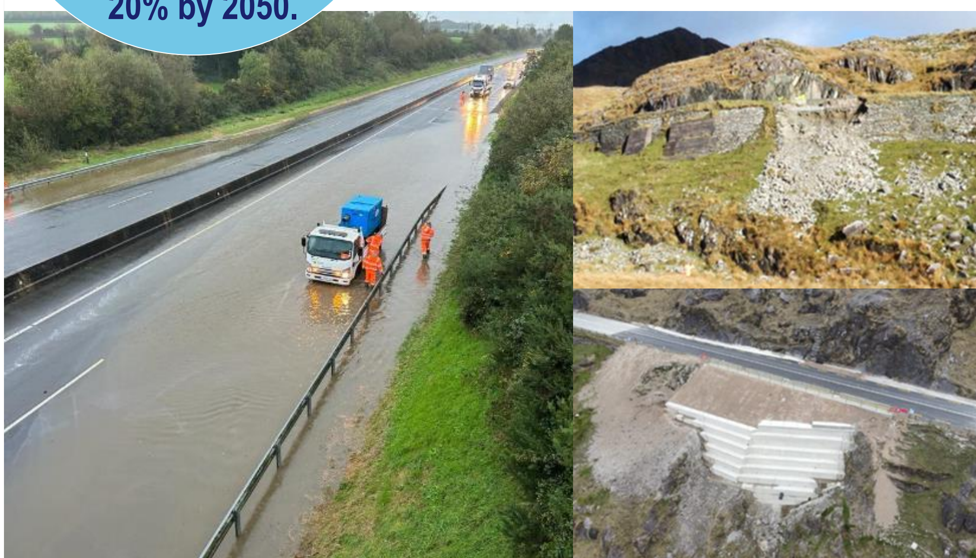
Recent weather-related incidents on the National Roads network, clockwise from left: Flooding on the M11, 2013; Landslide at Moll's Gap, 2016; Retaining walls works at Caha which failed in 2020 and were remediated in 2021
