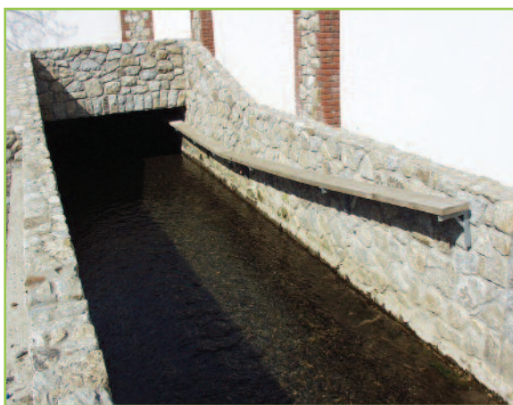
A culvert with an otter ledge attached on brackets. This section of artificial channel has a stonepitched base on which sand and gravel will lodge more readily than concrete.
