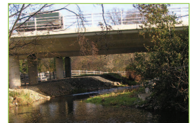
A well designed clear-span bridge retaining the existing river channel with piers set back from the river bank.
