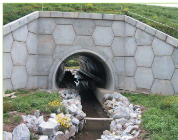
An example of a well designed oversized arched culvert with mammal ledges. The natural bed of this watercourse was maintained.
