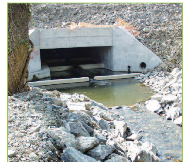
A well designed culvert which has a stepped profile to accommodate fish passage and an outlet pool to allow fish to pass upstream into the first of the steps. The culvert incorporates a cast mammal ledge.
