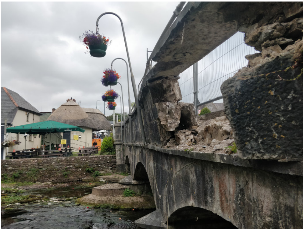
Figure 2: Damaged sections of the parapet to be repaired at Killeagh River Bridge (CC-N25-004.00).
