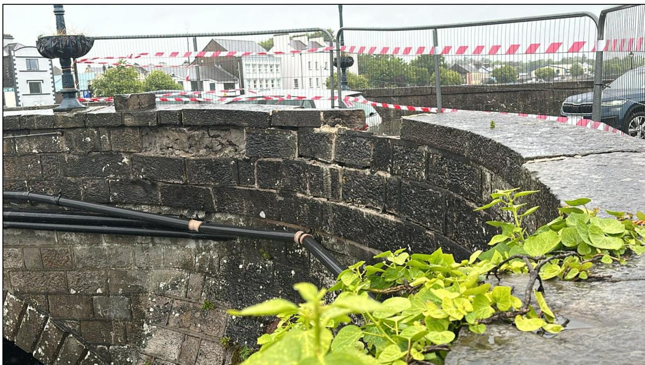
**Figure 3:** Damage to the riverside face of the parapet at Ballina Upper Bridge (MO-N59-001.70).
