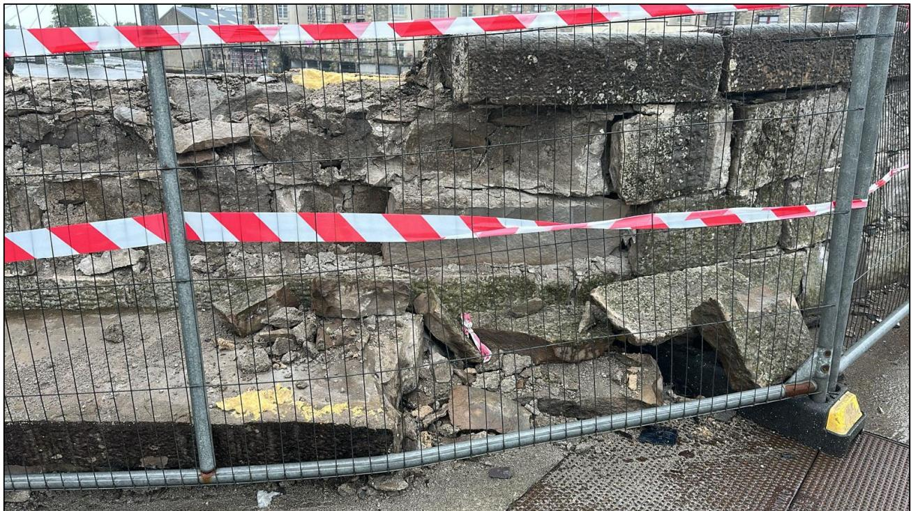
**Figure 2:** Damage to the roadside face of the parapet at Ballina Upper Bridge (MO-N59-001.70).
