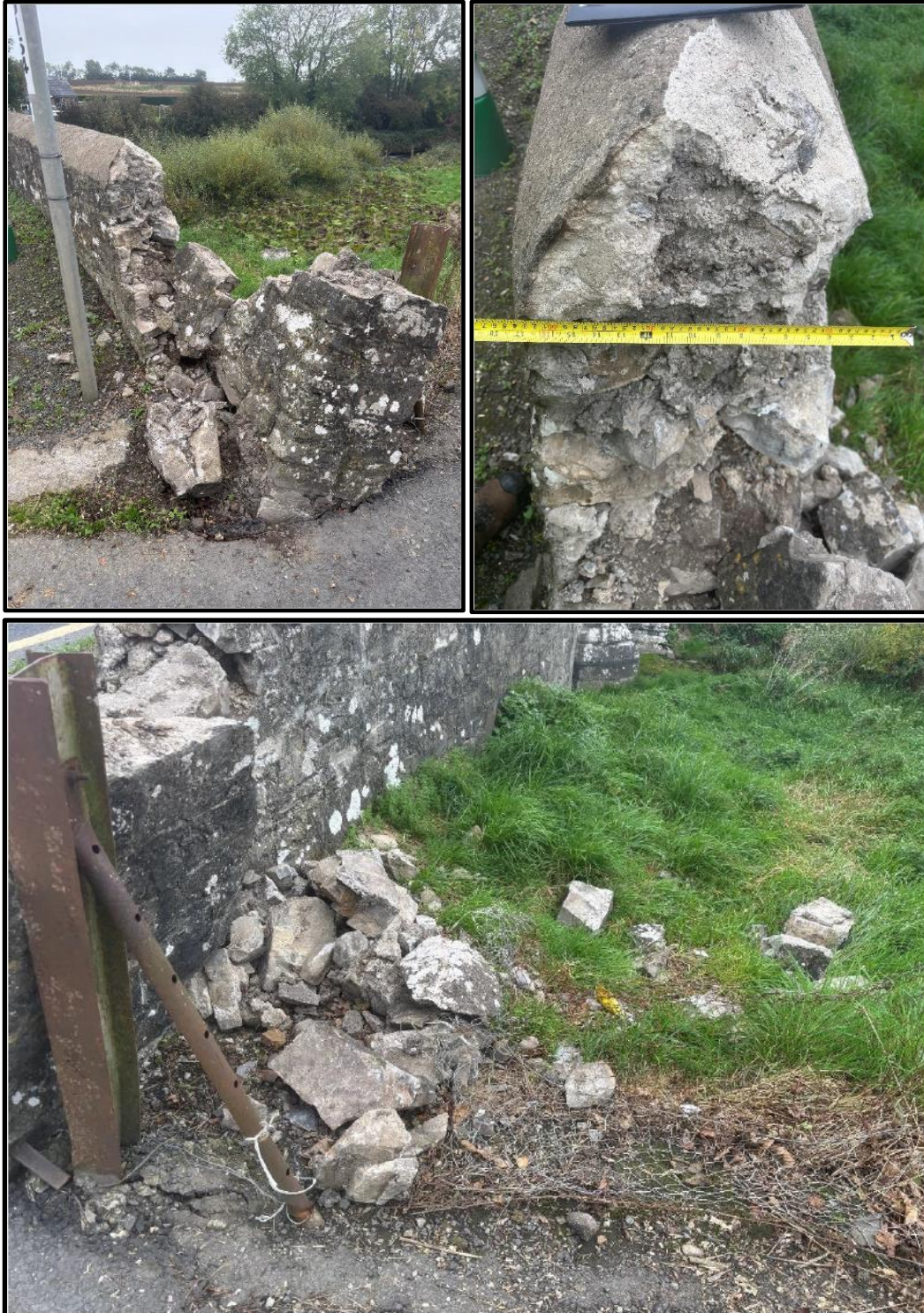
Plate 1 Damage to the eastern parapet and damaged mesh fencing (bottom only).
