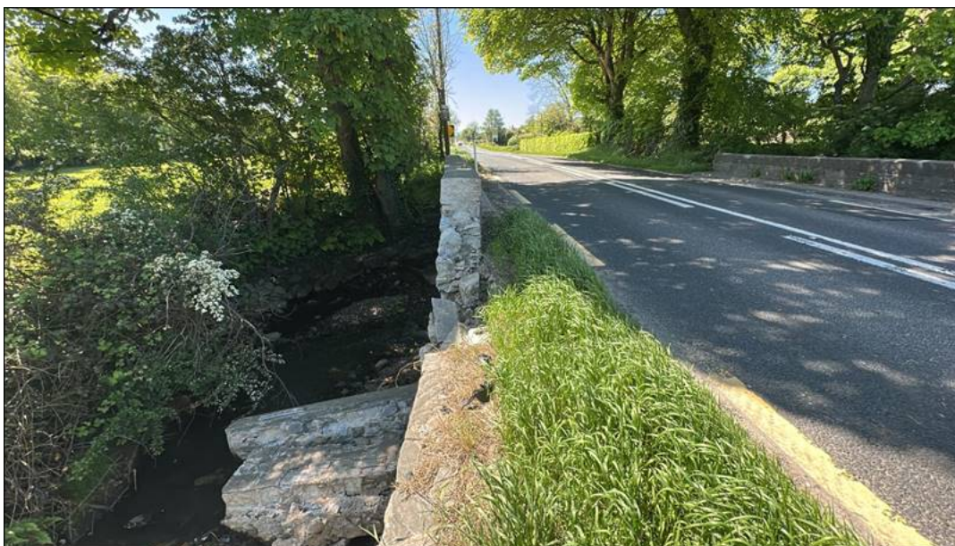
Figure 2: Damaged section of the parapet to be repaired at Mullandrait Bridge, with debris in watercourse (DL-N15-003.00).
