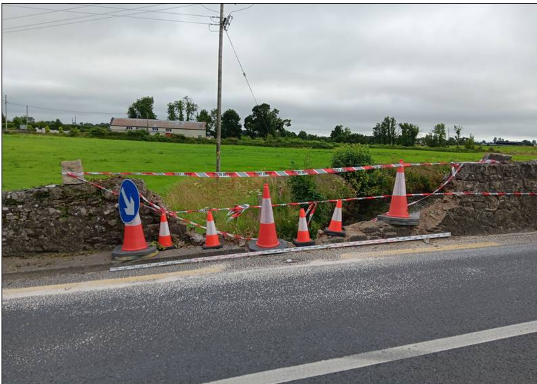
Figure 2: Damaged section of the parapet at New Bridge (GC-N63-013.00).
