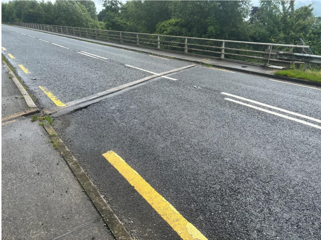
Plate 1 South expansion joint.
