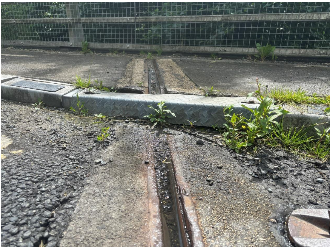
Plate 3 Galvanised steel kerb cover plate and expansion joint on footpath.
