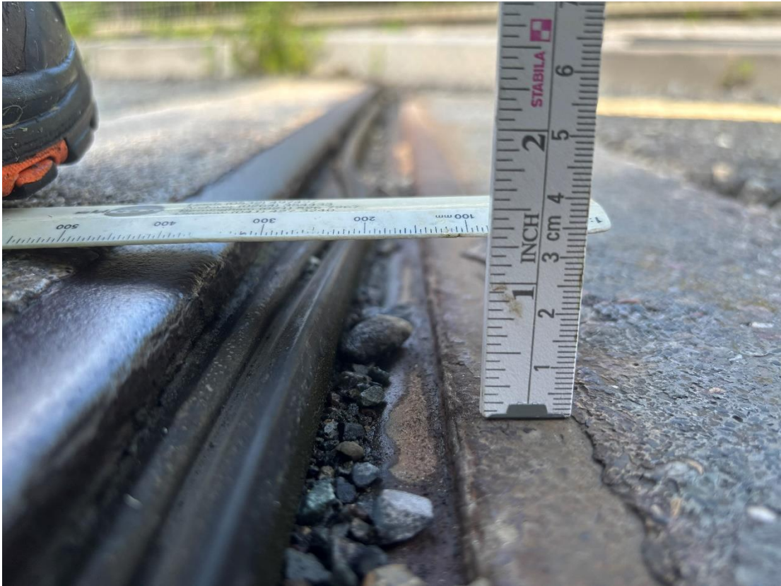
Plate 4 Maximum settlement on the north expansion joint.
