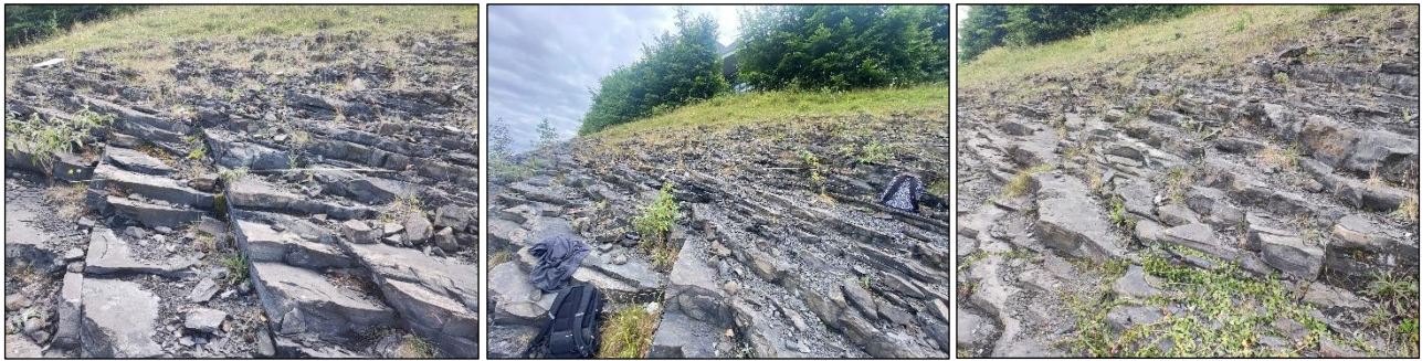
Figure 75 Photographs of the studied rock face at the Liffey Valley site.
