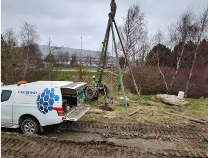
Figure 100 Cable percussion borehole set up.
