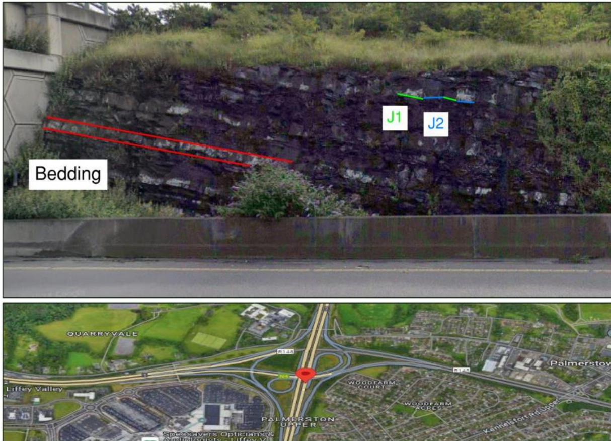
Figure 68 Exposure of Calp Limestone encountered along the main carriageway at Junction 7 of the M50 motorway during the virtual site walkover.
