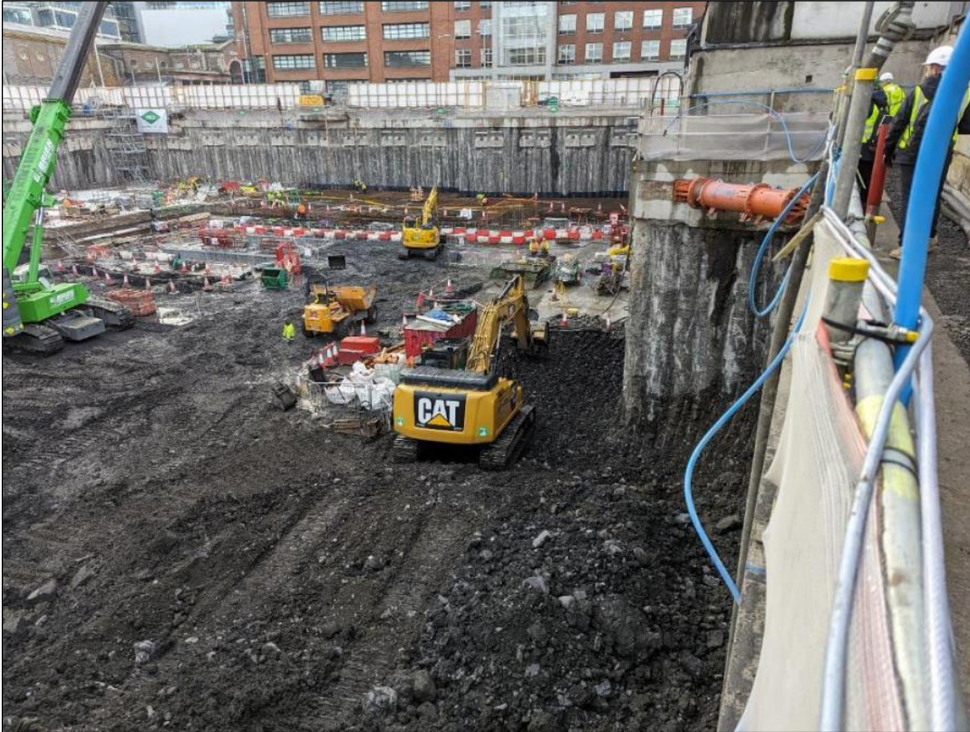
Figure 70 Overview of excavation, looking north.
