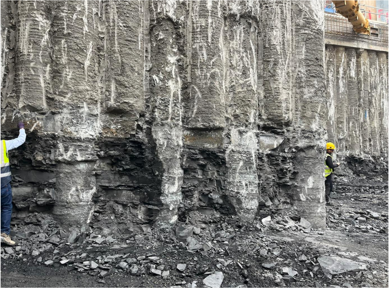
Figure 87 Calp Limestone exposure at the One Adelaide Road site.
