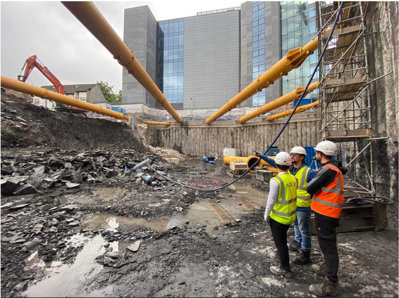
Figure 89 Surface of excavation at the One Adelaide Road site.
