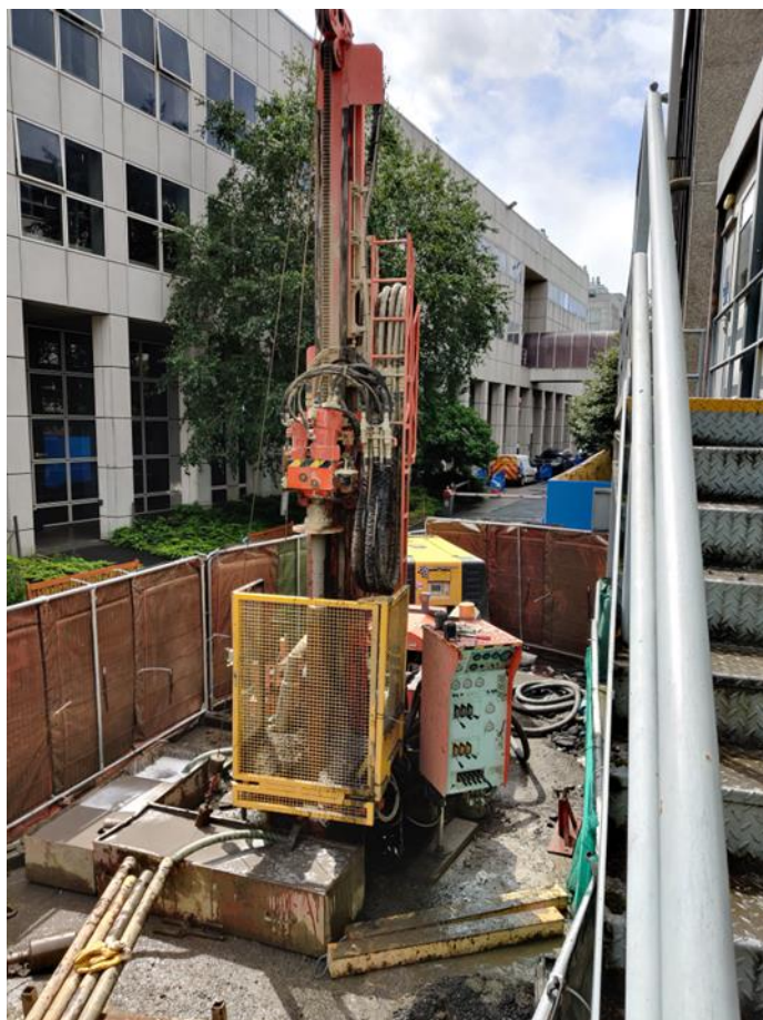
Figure 102 Geobore-S in use in urban environment.
