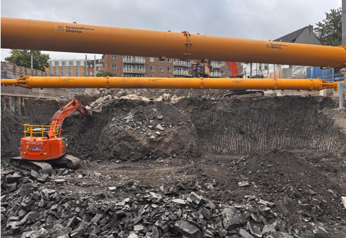
Figure 85 Photograph of the face of the excavation.
