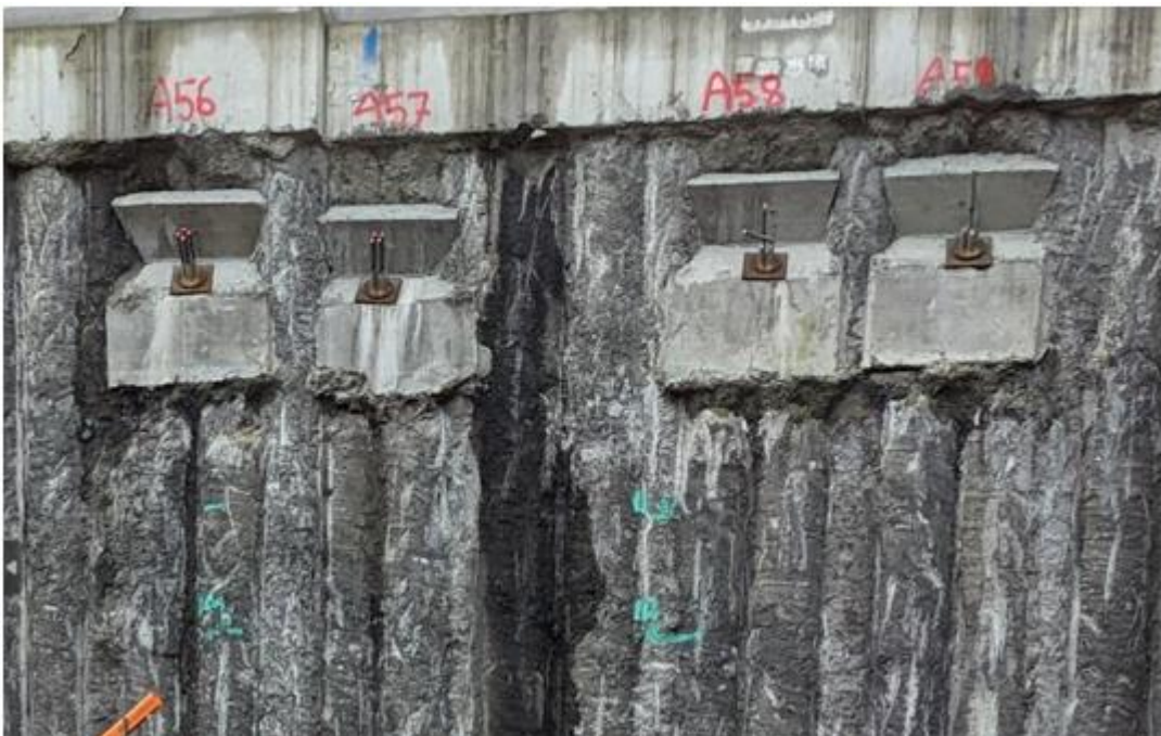
Figure 71 Soft-soft-hard wall with anchors, eastern side of the site.
