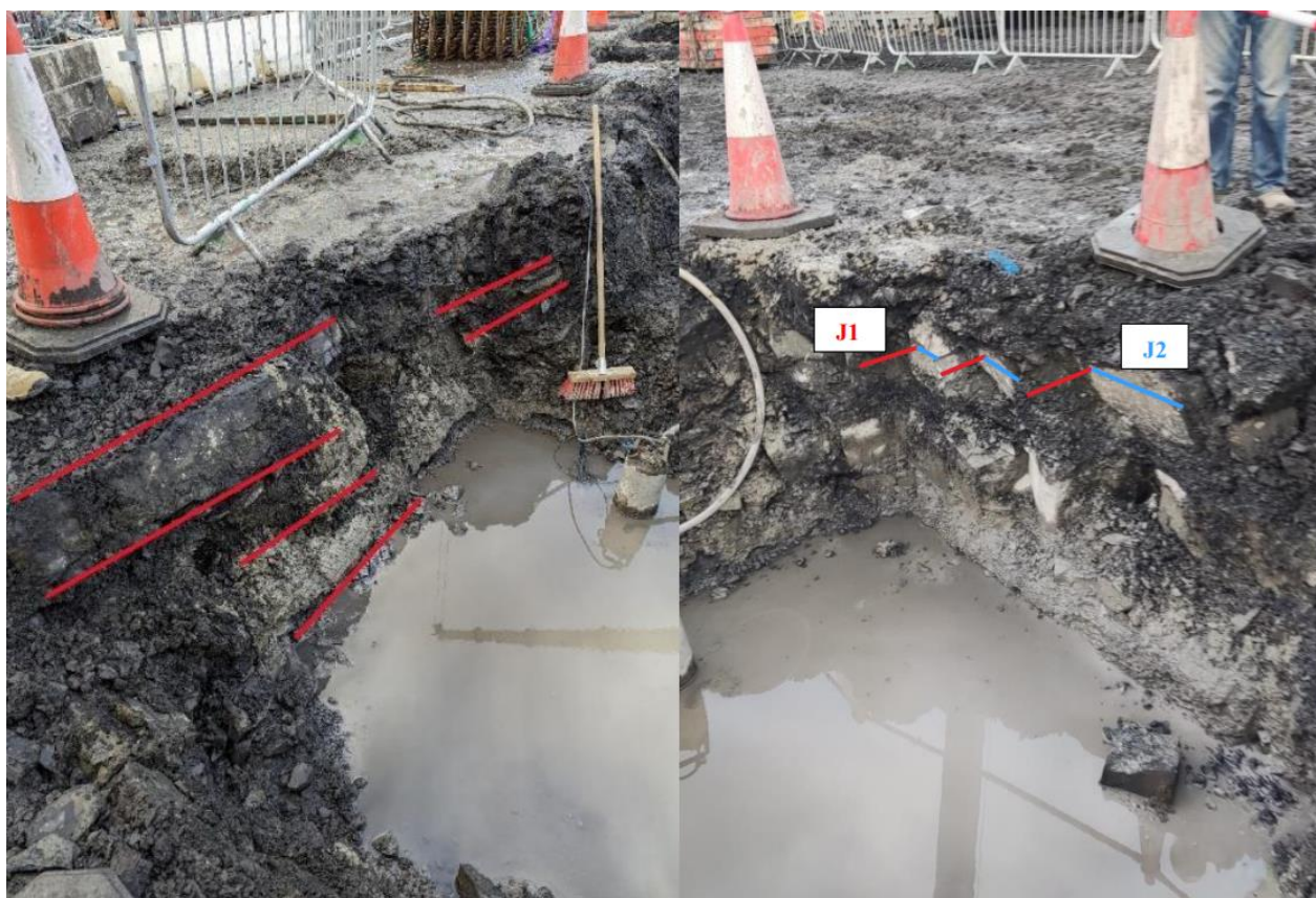
Figure 72 On the left Image looking north-east into lift pit excavation and on the right Image looking northwest of lift pit excavation depicting the subvertical joints.
