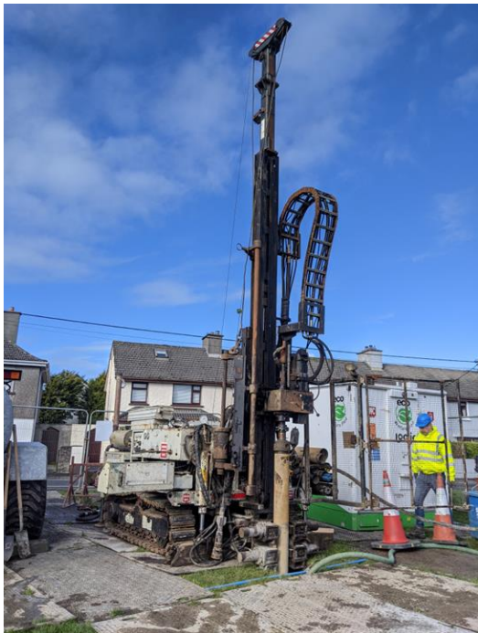
Figure 101 Rotary drilling in residential/urban environment.
