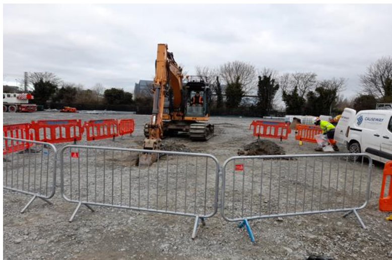
Figure 99 Trial pitting with protective fencing in place as a health and safety measure.
