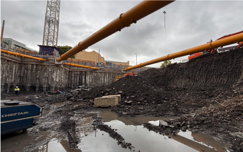
Figure 86 Photograph showing the vertical faces of the excavation and the bedrock exposure at distance.
