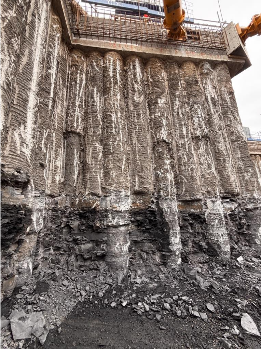
Figure 88 Calp Limestone exposure at the One Adelaide Road site.
