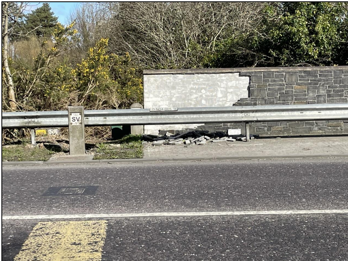
Plate 1 Northern parapet with missing cladding on the eastern end of the parapet.
