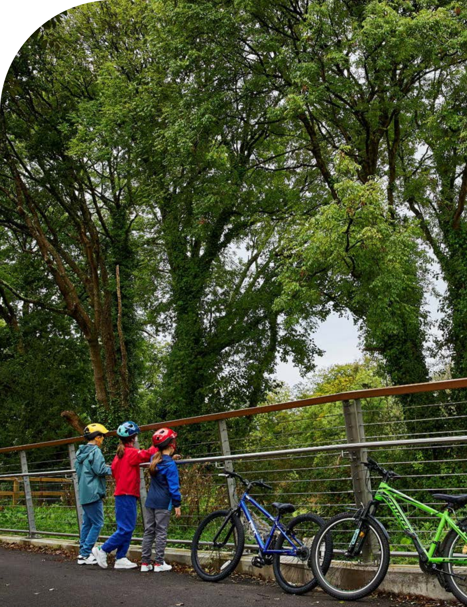
Windblade Bridge on the Midleton to Youghal Greenway, Cork
