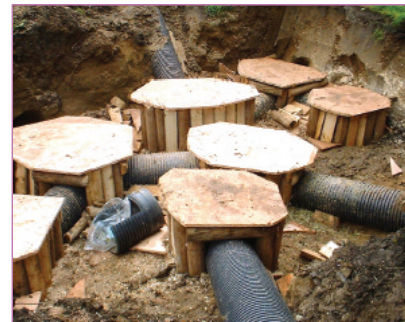
An example of an artificial sett under construction, with pipe tunnels and eight chambers.
