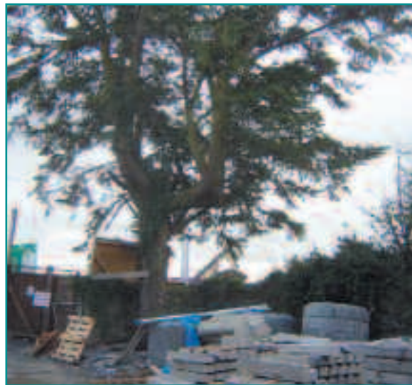
Unprotected tree. Note the storage of materials around the RPA. This tree will eventually succumb to the effect of soil compaction.
