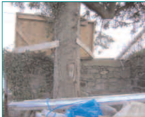
Tree displaying bark damage as a result of no protection. Possible entry point for pathogens.
