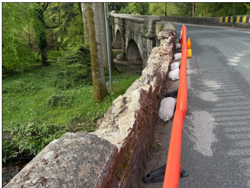
Plate 1 – View south towards Lismore Bridge 2 (WC-N72-001.00).
