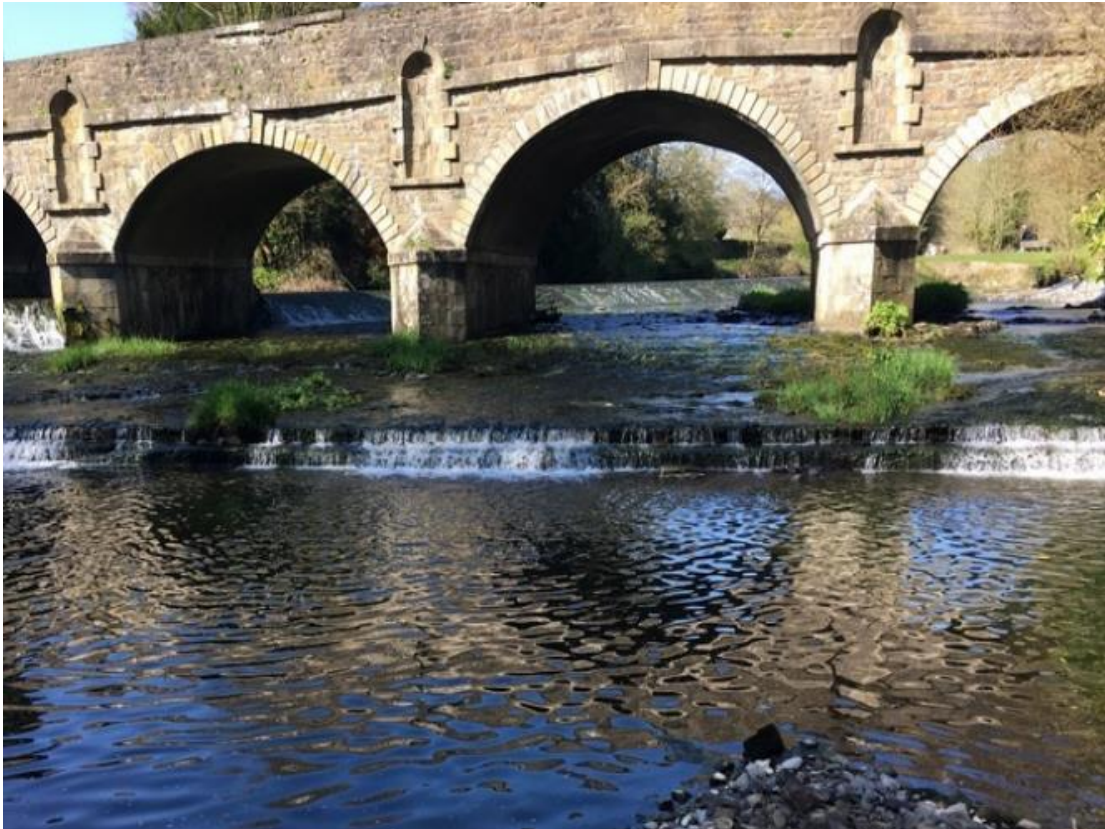
Plate 6 Downstream of bridge showing masonry apron.
