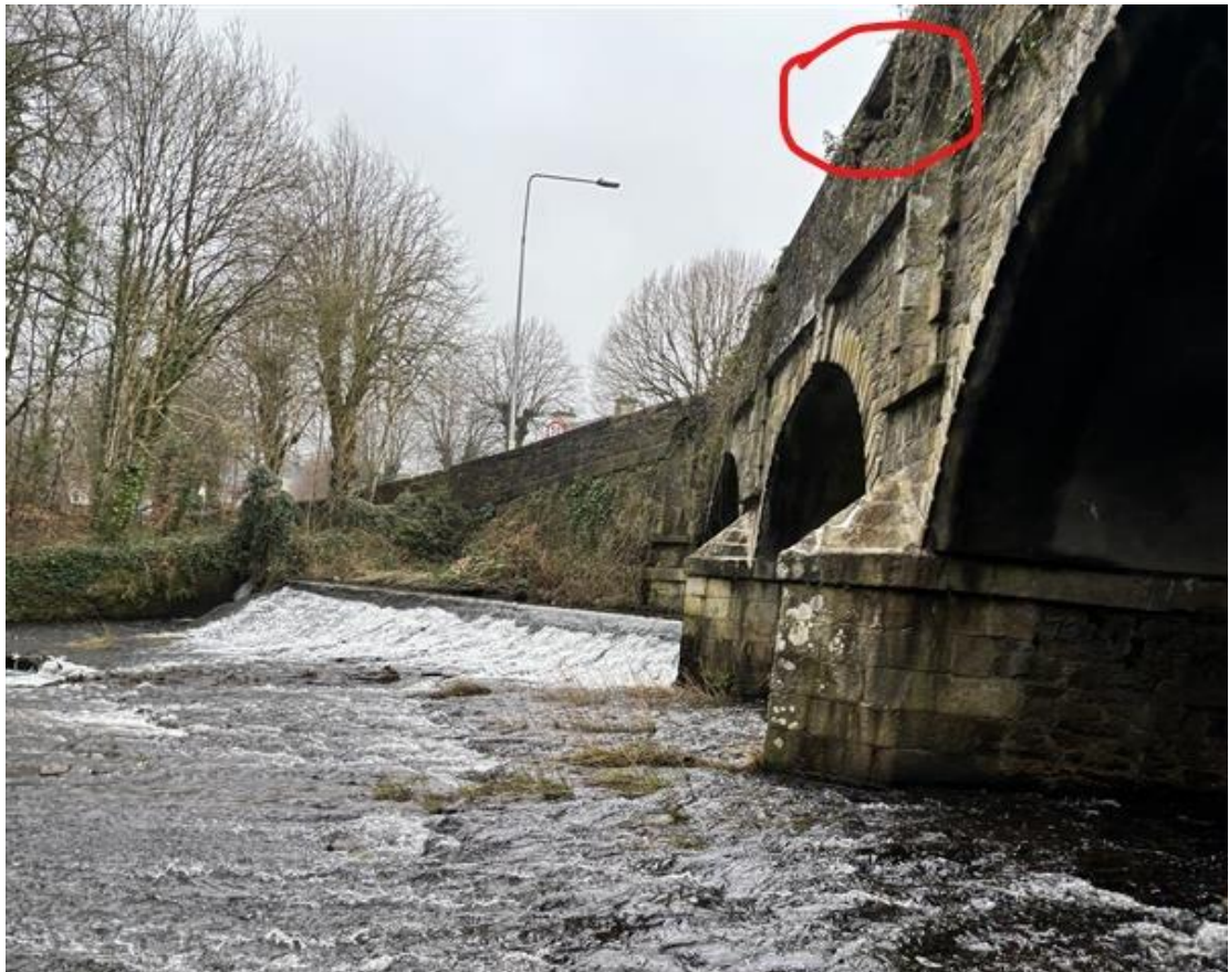
Plate 4 Castlecomer Bridge with damage to southern parapet circled in red.
