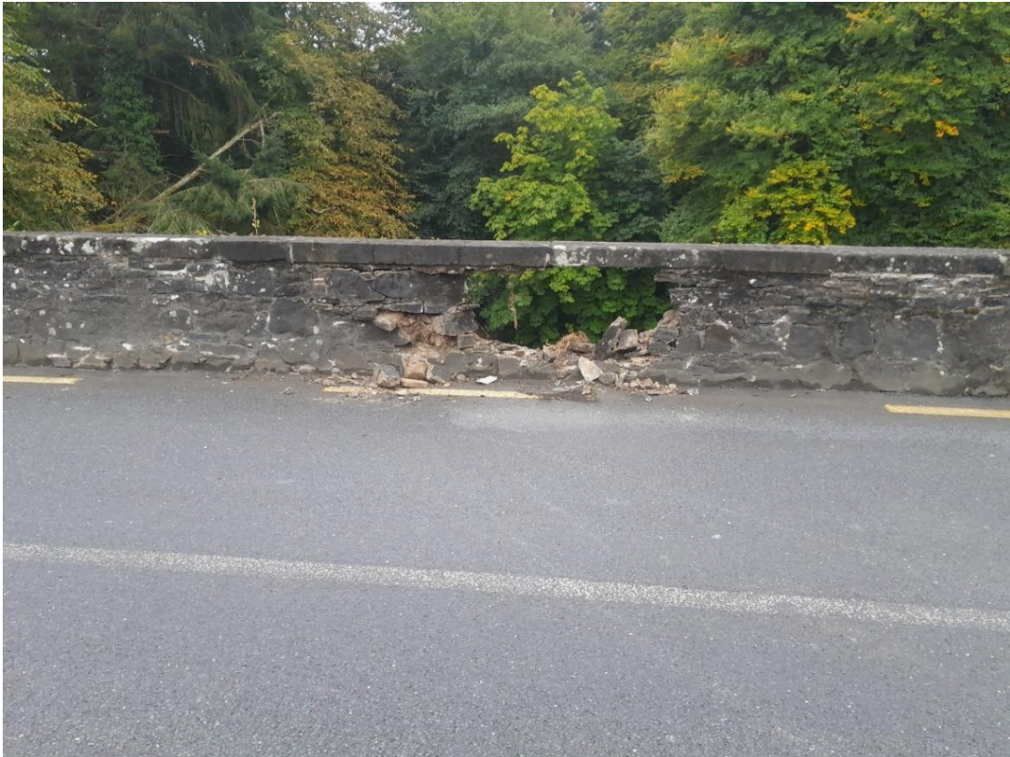
Plate 2 Southern parapet with damage resulting from vehicle strike.
