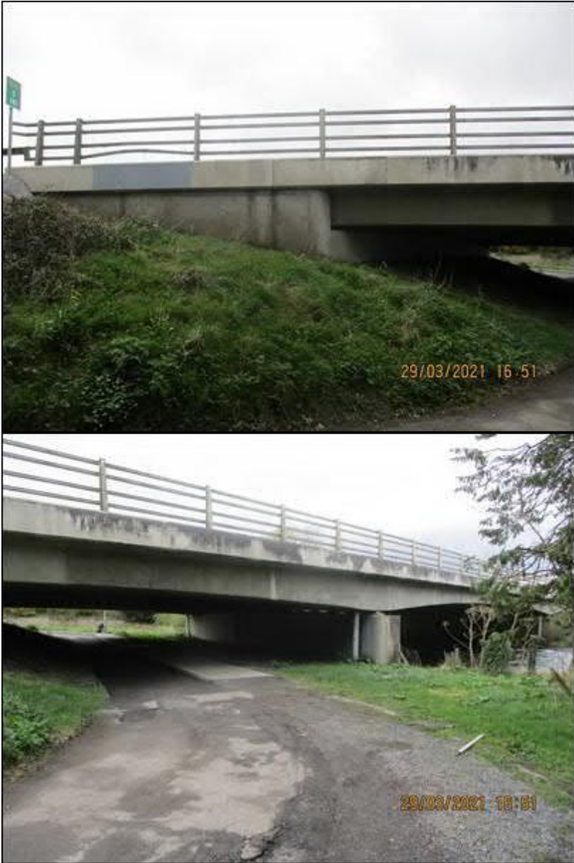
Plate 1 Location of works area (left) and adjoining road (right).
