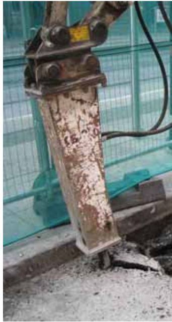
Plate 2: View from northeast of mechanical excavation of permanent road surface
