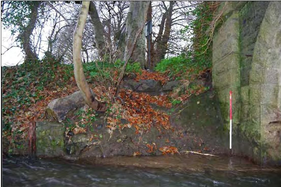
**Plate 82:** North-facing view showing concrete underpinning of upstream side of Balheary Bridge and section of masonry wall (Feature 4) located to right of picture, on north side of the Ward River (1m scale).
