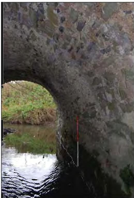
**Plate 46:** West-facing view of intrados on north side of **Arch no. 4**, showing bulge located across the arch-ceiling of the phase 1 mid-section, Lissenhall Bridge, Feature 1 (1m scale).
