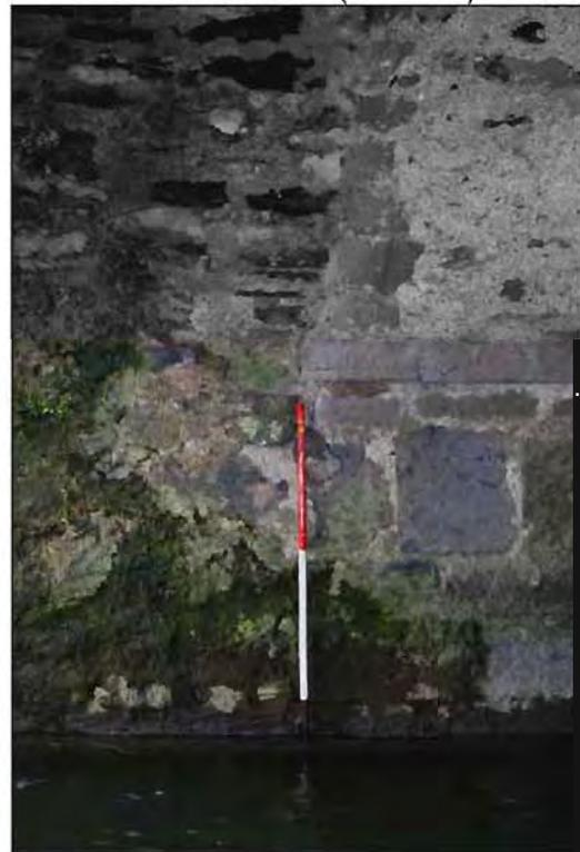
**Plate 22:** Transition-point between mid-section (Phase 1) and upstream section (Phase 2), north side of **Arch no. 2** (1m scale).
