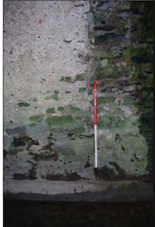
**Plate 20:** Transition-point between mid-section (Phase 1) and upstream section (Phase 2), north side of **Arch no. 1** (1m scale).
