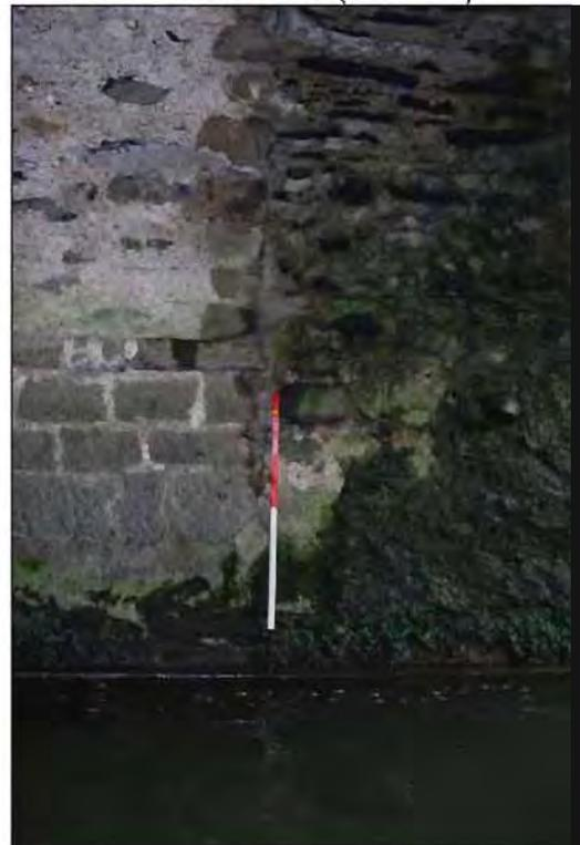
**Plate 34:** Transition-point between mid-section (Phase 1) and downstream section (Phase 2), north side of **Arch no. 3** (1m scale).
