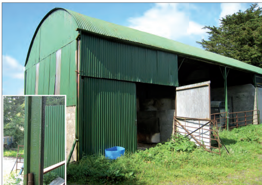
Typical 1960s barn in County Tipperary, with a framing of reused running rails. Inset: the inscription reads 'G.N.R.Co Ireland', indicating that the rails were manufactured for the Great Northern Railway Company.
