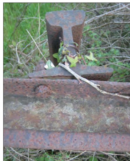
Details of running rail crash barrier.
