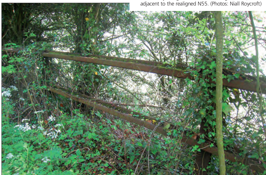
Railway running rails reused as crash barrier on top of Dundavan Bridge (South).
