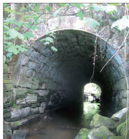
The culvert under the road embankment adjacent to Dundavan Bridge (North).
