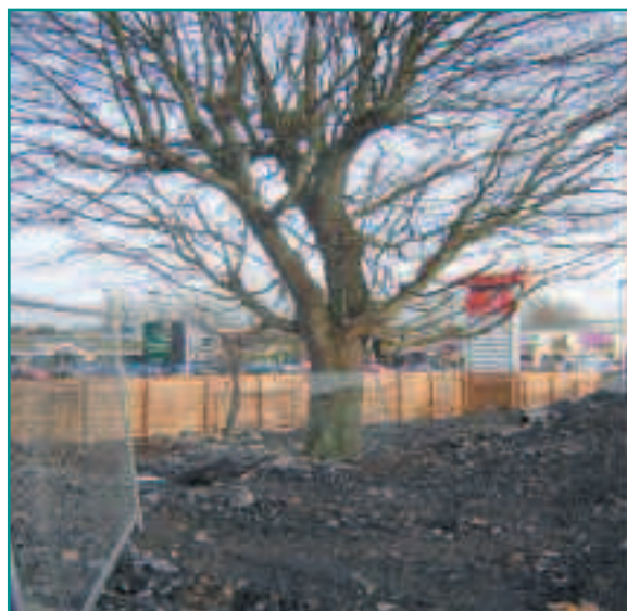
An example of an unprotected tree where ground levels have been altered.
